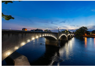
Gillett Pedestrian Bridge
