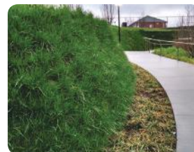
⑤ Reinforced earth / green wall
