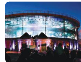
④ Repurposed water tank
