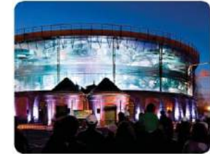
④ Repurposed water tank
