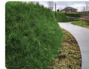
⑤ Reinforced earth / green wall
