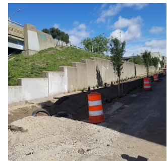
Retaining wall Ionia/Wealthy St. SW
