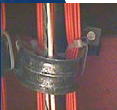
Figure 37. Example of a common cause of a fiber failure
