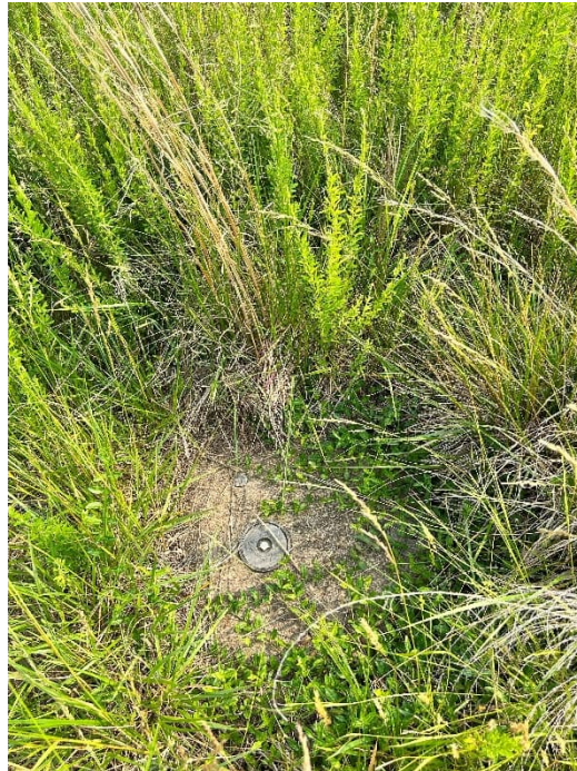
Photograph 13. Typical flush mount monitoring well with T-bar for locating.
