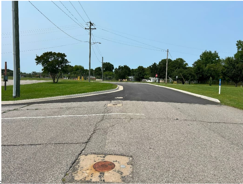
Photograph 23. Paved section of N. 4 th St with concrete curbs installed at northeast corner of Bldg. 66.
