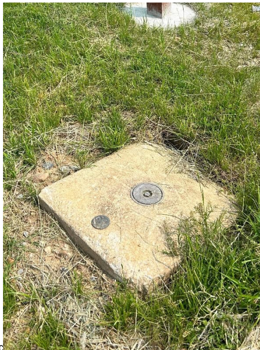
Photograph 30. OU8-MW-53 disturbed during construction activities, concrete pad reset in correct location over casing FY24.
