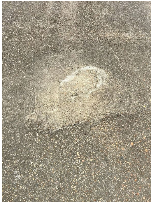
Photograph 28. Abandoned monitoring location in concrete during the network optimization activity.
