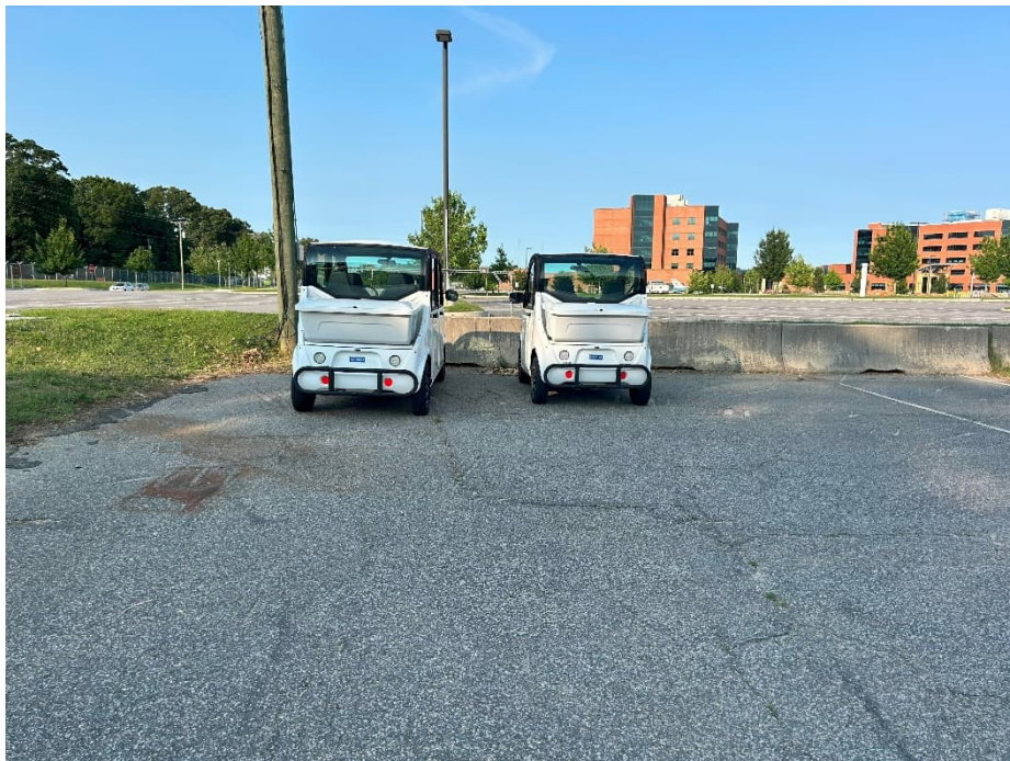
Photograph 2. View of east side of PX Gas Station looking east-northeast, shows new parking lot.
