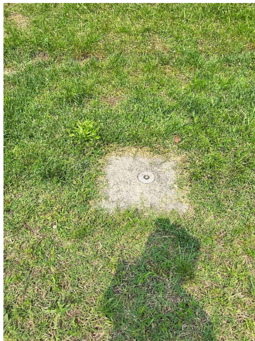
Photograph 6. Typical flush mount monitoring well in grass.
