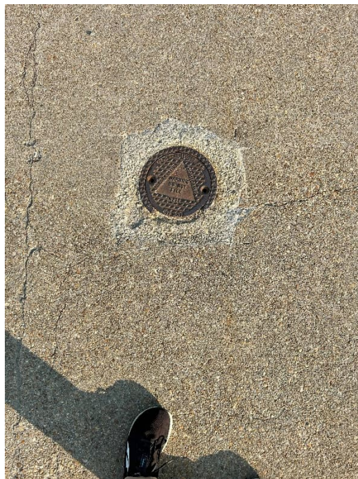
Photograph 6. Typical flush mount monitoring well.
