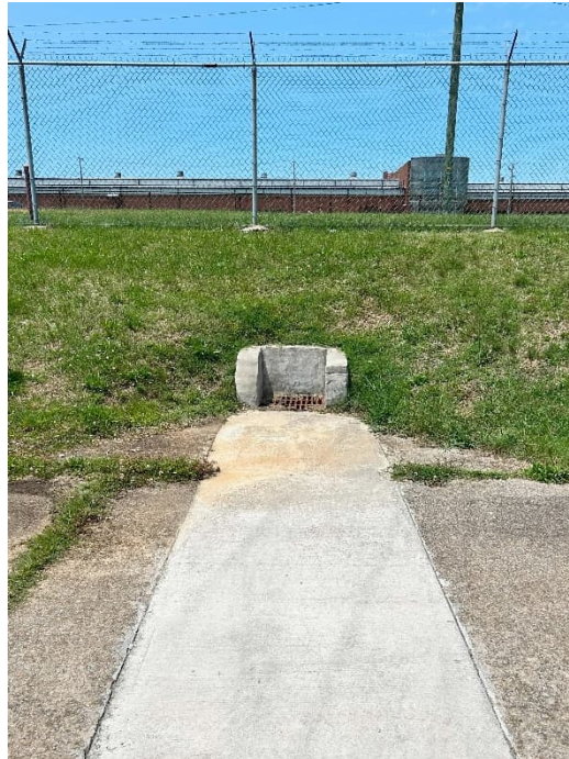
Photograph 3. Storm drain west of Bldg. 151; repaired as part of larger sewer repair work done around DSCR in FY24.
