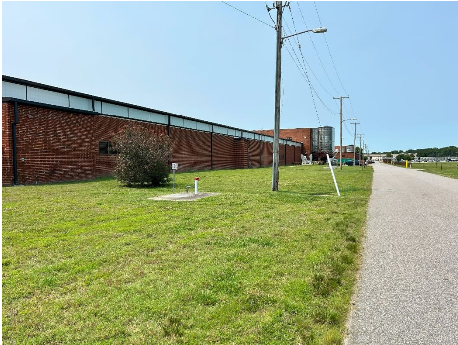
Photograph 3. View of OU 1 eastern edge looking north from southeast corner of the site.
