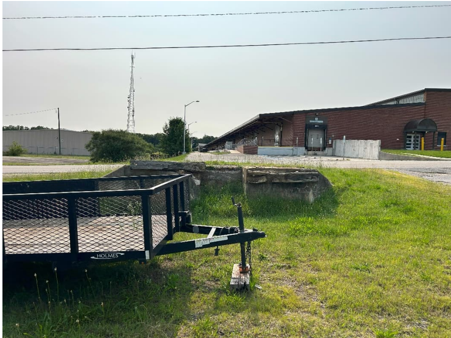
Photograph 17. Damaged rail stop.
