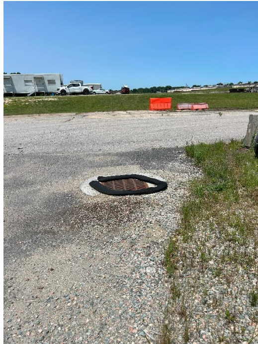
Photograph 14. Storm drain repair in northern area of OU 1 completed FY24.
