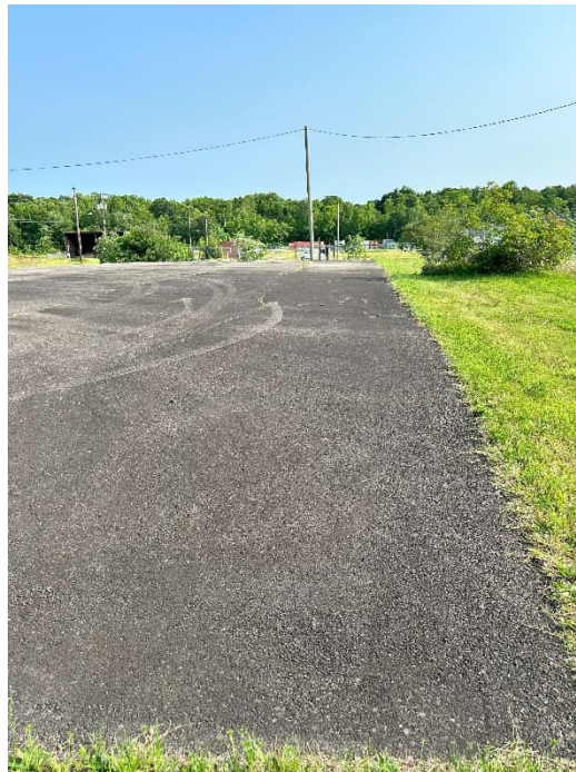
Photograph 4. West side of OU 12 cap looking south.
