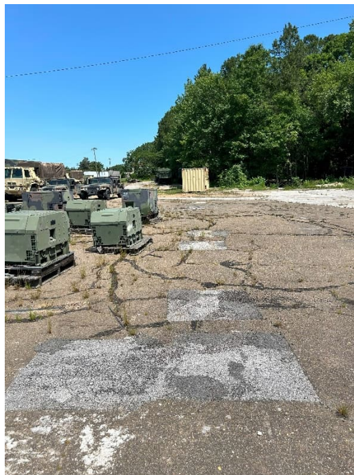
Photograph 14. Abandoned well pads in asphalt during the network optimization activity in FY23.
