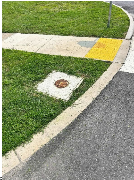
Photograph 25. MWANP-26, replaced concrete pad due to Construction of Intersection of G Road and N 4 th St in FY24.
