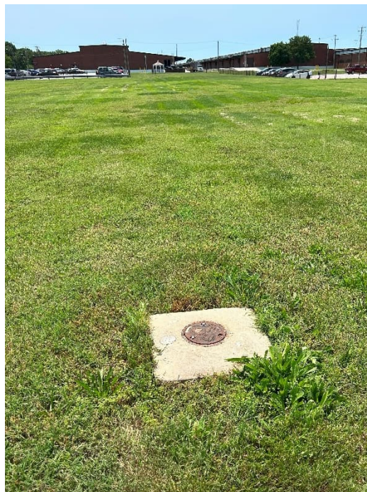
Photograph 8. View of MW-96, well pad settling repaired in September 2024.
