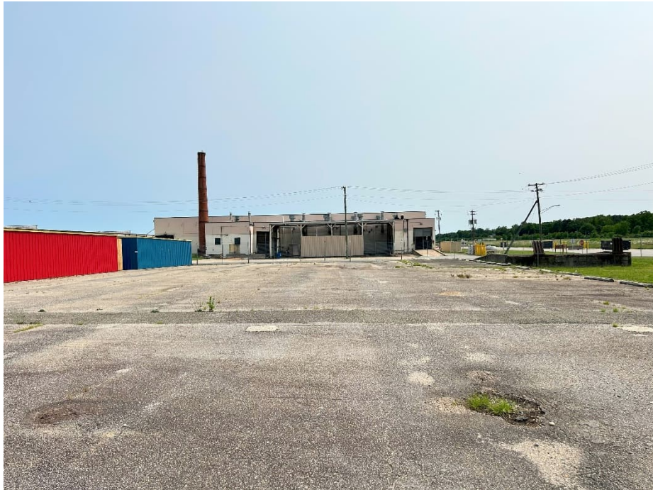
Photograph 11. Looking south at Bldg. 65 in parking lot with deteriorating asphalt.
