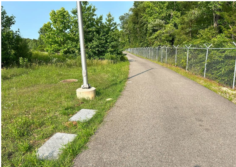
Photograph 20. Looking east along Perimeter Road, new streetlamp installed FY24.
