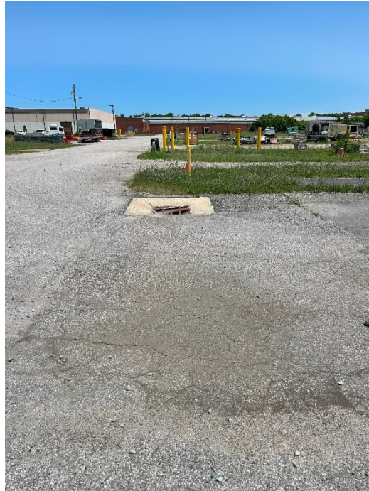
Photograph 13. Northern part of OU 1, typical completed storm drain.
