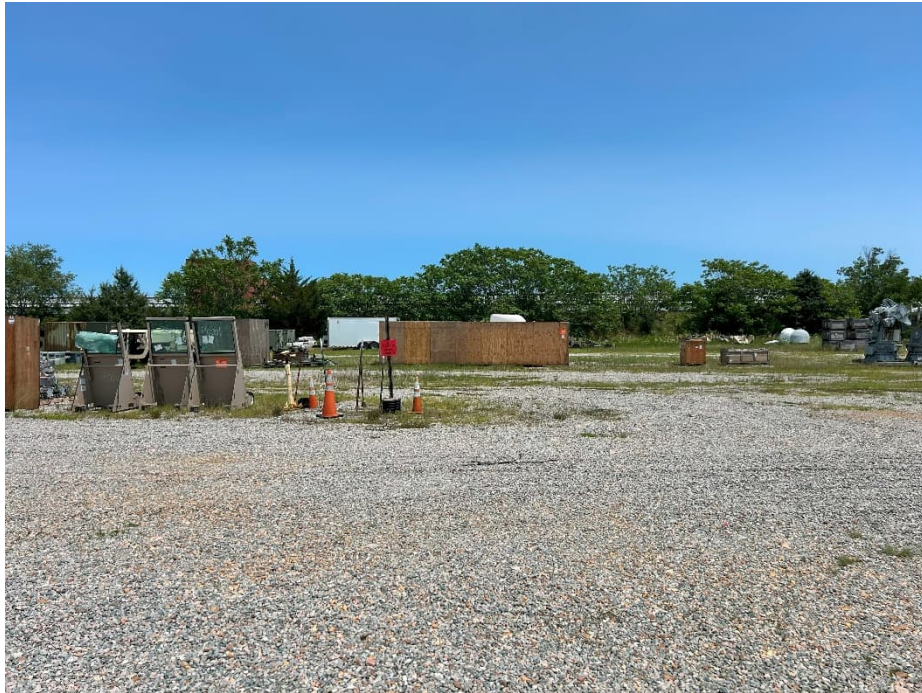
Photograph 11. View of area previously marked as and used for concrete washout.
