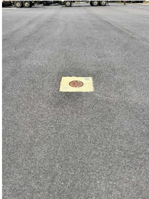
Photograph 25. Repaired well pad in northern asphalt repair area in FY24.
