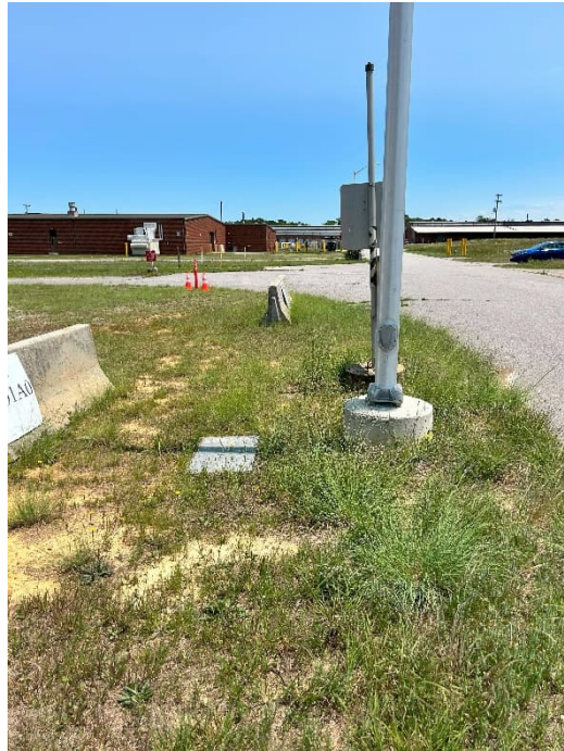
Photograph 27. New lamp post, looking towards Bldg. 40.
