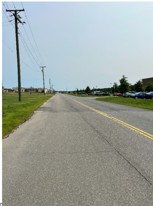
Photograph 22. C Road, looking South at repaved section in FY24, approximately 800 ft to intersection with N. 4 th St.
