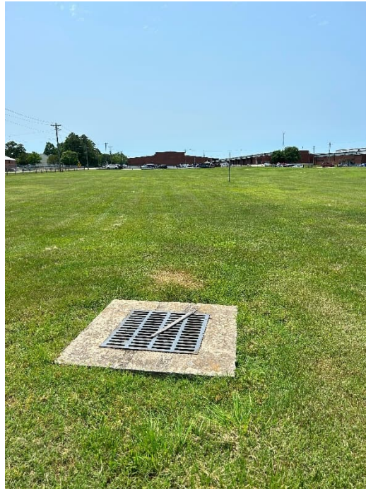
Photograph 5. View of typical OU 2 storm drain; no signs of erosion or sedimentation.
