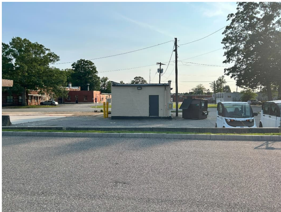
Photograph 4. North end of PX Gas Station looking west-southwest.
