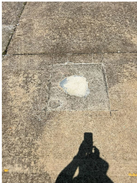
Photograph 30. West side of Bldg. 54 with abandoned monitoring location during network optimization activity.
