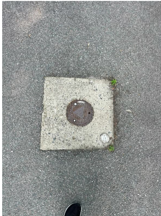
Photograph 10. Typical flush mount well completion in asphalt, Perimeter Road.
