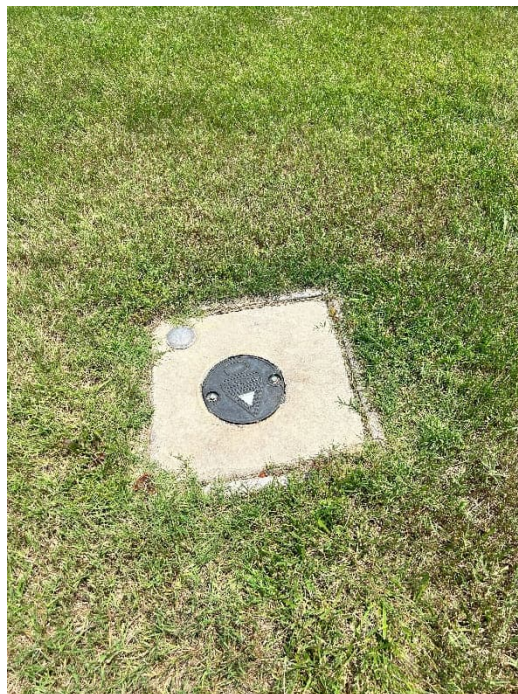
Photograph 4. View of typical OU 2 flush mount well completion.
