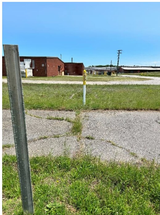
Photograph 28. Above ground markers installed denoting the location of a gas line.
