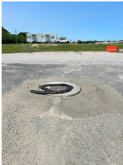
Photograph 14. Storm drain repaired in northwestern area of OU 1 during FY24.
