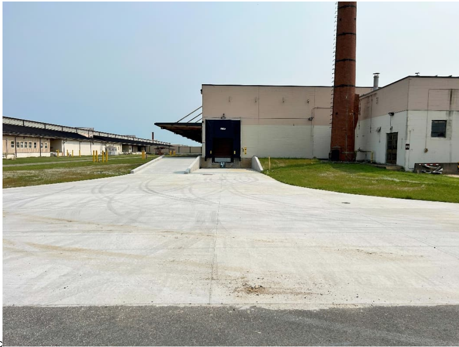
Photograph 27. Completed loading dock construction at northeast corner of Bldg. 65.
