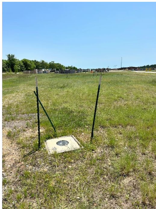
Photograph 18. View of typical flush mount completion in open storage area, installed in 2021.
