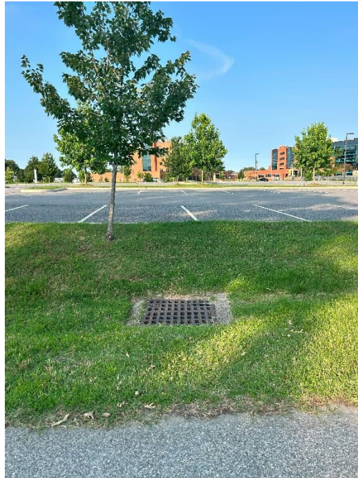
Photograph 3. PX Gas Station storm drain; no new erosion or sedimentation visible.
