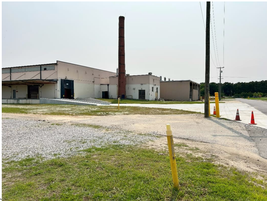
Photograph 26. Restored staging area of construction activity at northeast corner of Bldg. 65.
