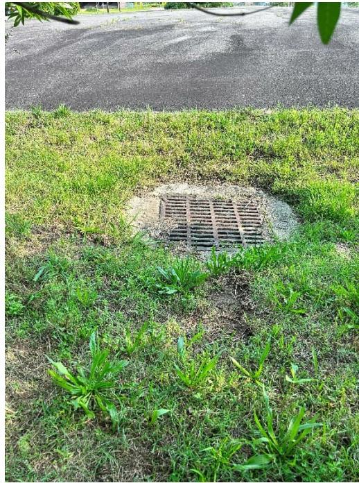
Photograph 3. View of OU 12 cap looking south. No erosion or sedimentation are visible at storm drain.
