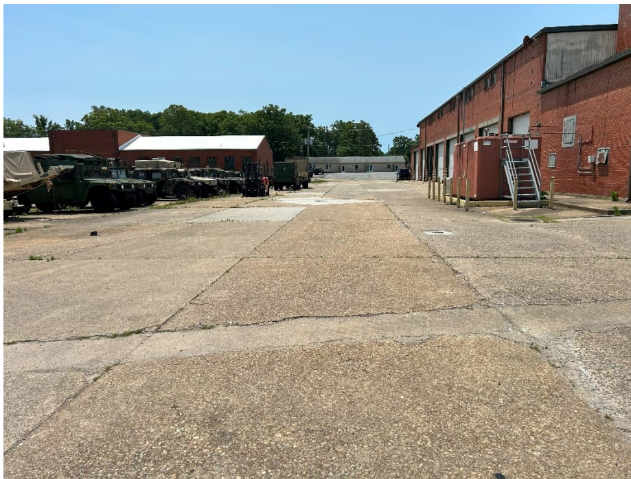
Photograph 12. View of OU 3 looking south from north of Bldg. 151.
