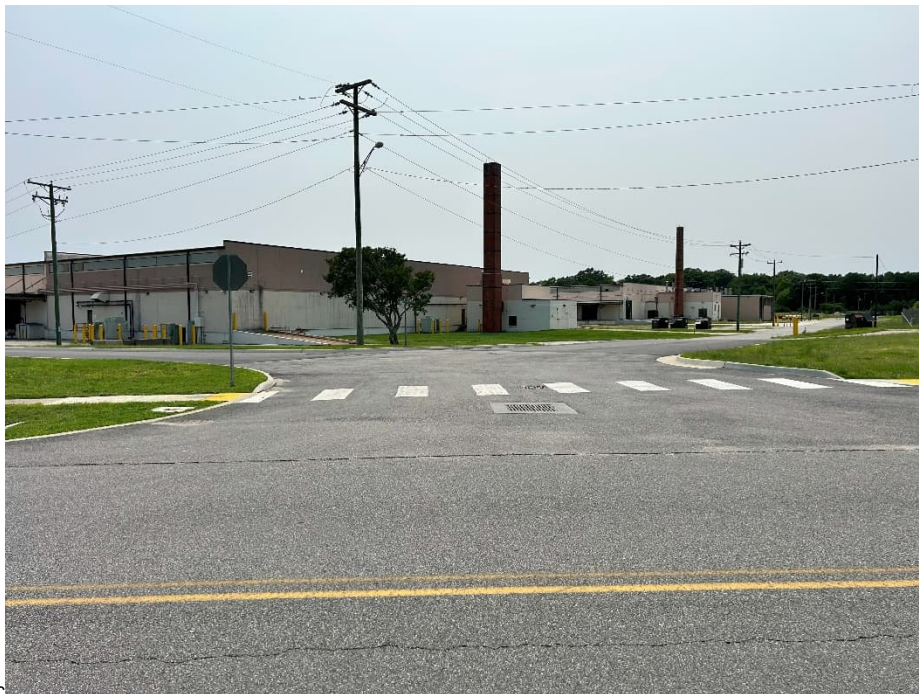
Photograph 24. Looking east at new intersection constructed at G Road and N. 4 th St.
