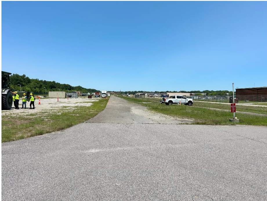
Photograph 4. View of laydown area west of Bldg. 40, fresh crush and run base material visible.
