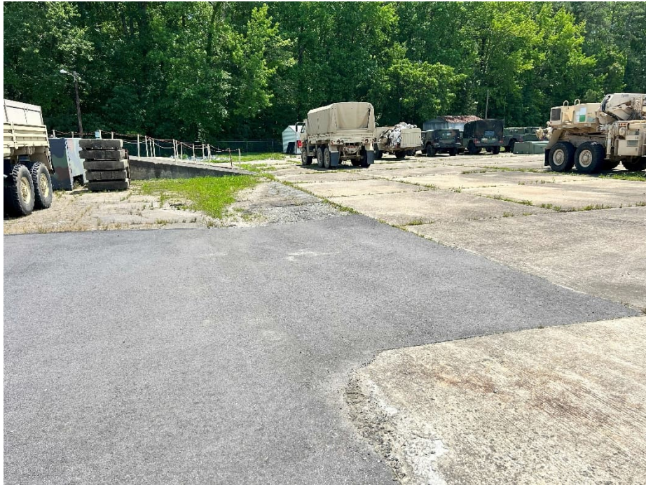
Photograph 7. Southeast corner of previously repaired northern asphalt area.
