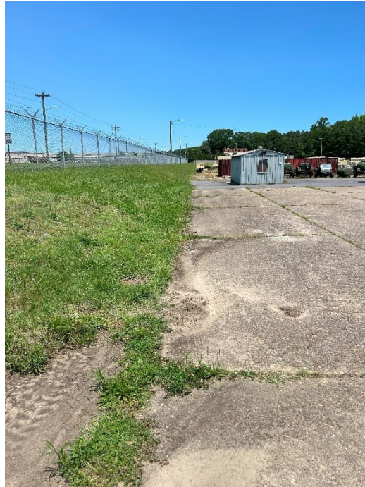
Photograph 5. View of OU 3 looking north from the west side of Bldg. 140.
