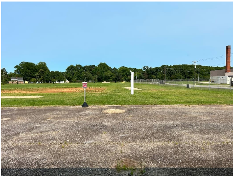
Photograph 10. Looking east towards ball field at southern end of parking lot in OU with deteriorating asphalt.
