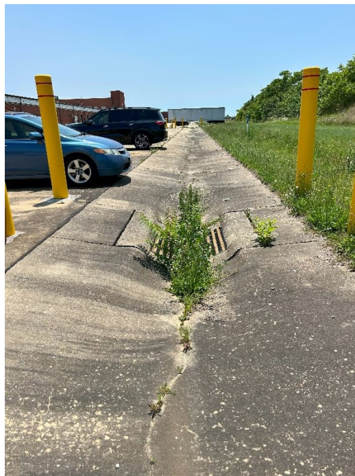
Photograph 20. Drainage ditch west of Bldg. 54 with vegetation.
