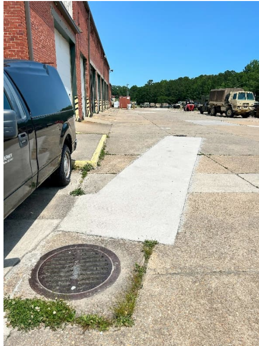
Photograph 13. View of OU looking north from south of Bldg. 151.
