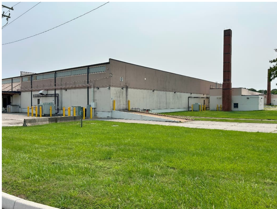
Photograph 14. View of northeast corner of Bldg. 66 where southern pump test was located.
