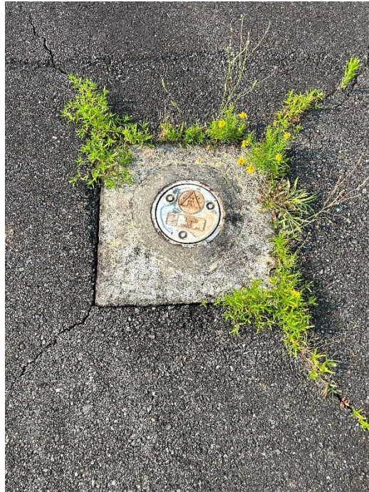
Photograph 7. OU 12 typical flush mount monitoring well.
