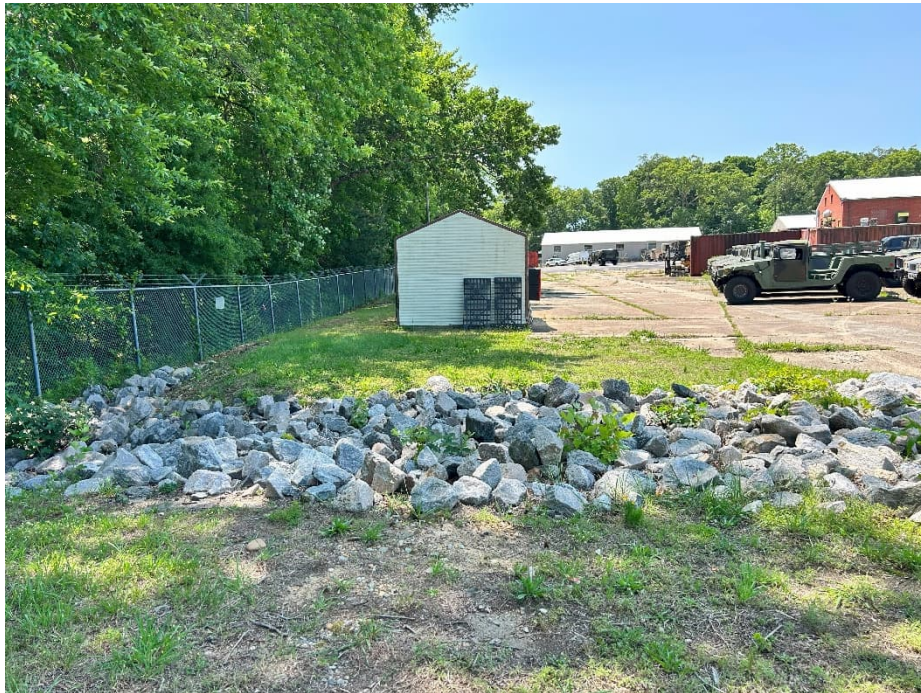
Photograph 10. View of OU 3 drainage basin with riprap to eliminate erosion.
