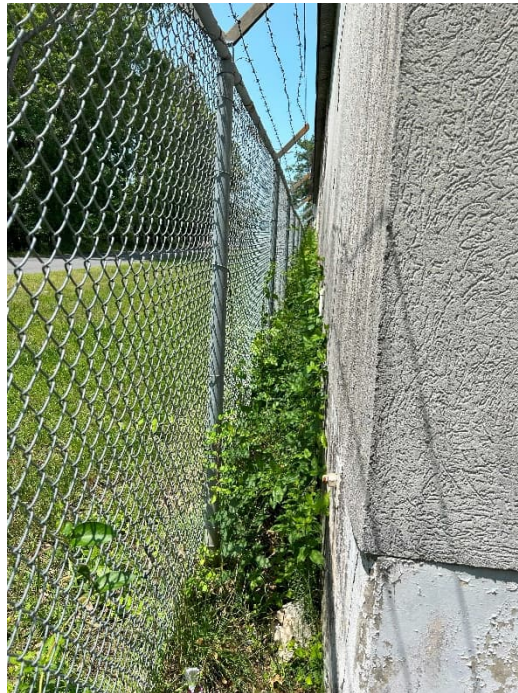
Photograph 22. Vines growing on perimeter fence along Alcott Road.
