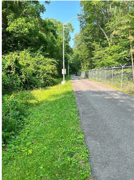
Photograph 21. Looking east, Perimeter Road, new street lamps installed FY24.
