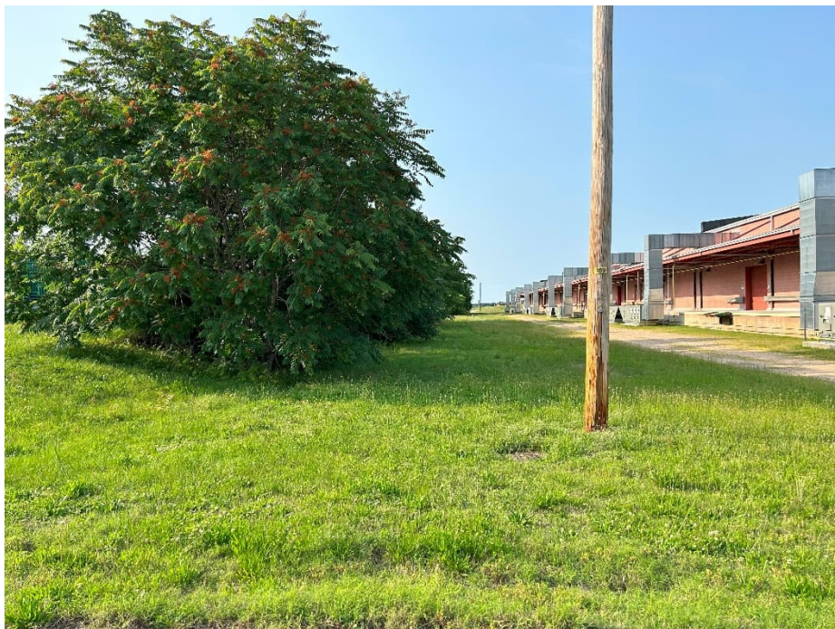
Photograph 6. Southeast corner of OU 11 looking northwest.
