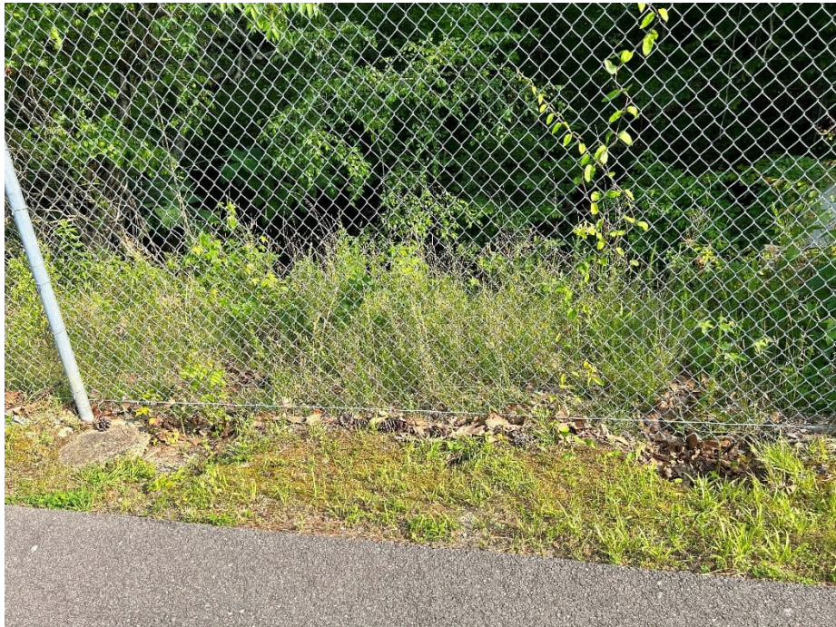
Photograph 2622. Animal burrows under fence at Kingsland Creek near intersection of G Road and Perimeter Road.
