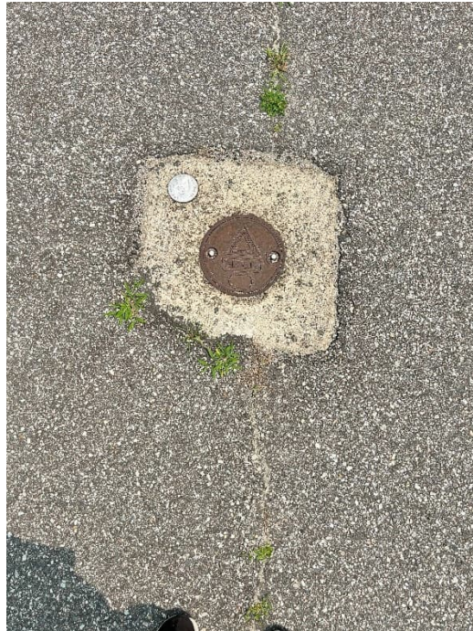
Photograph 5. View of typical flush mount well completion in asphalt.
