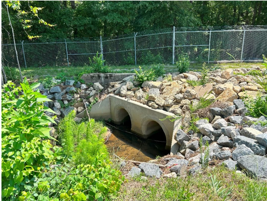
Photograph 27. Repaired fence section and repaired pass through of No Name Creek to the wooded area.
