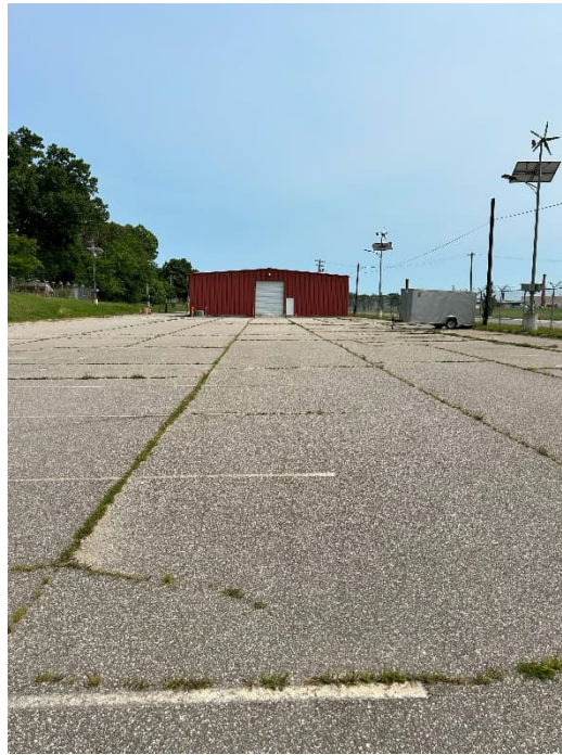
Photograph 3. View of the west side of Dervishian ARC looking south.
