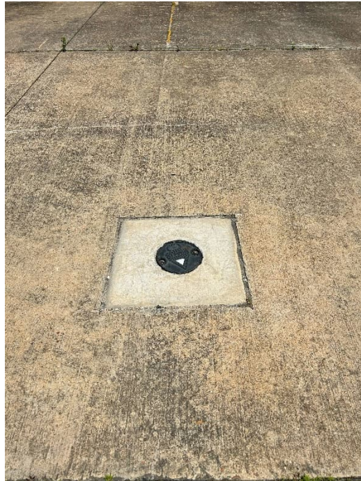
Photograph 19. View of typical flush mount completion in concrete, installed in 2021.
