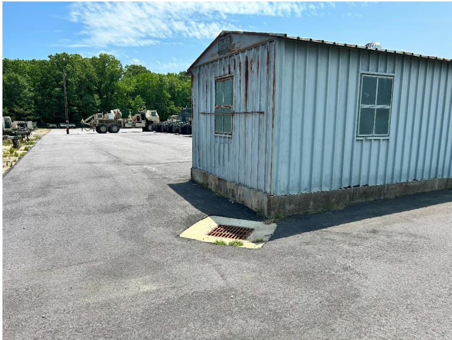
Photograph 24. Northwest corner of repaired northern asphalt area.
