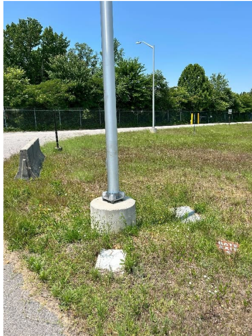
Photograph 25. Streetlamp installed in 2022, surface disturbance no longer visible.
