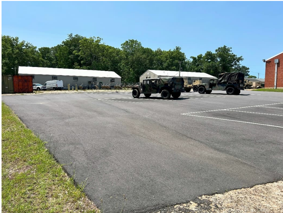
Photograph 16. Northeast corner of southern repaired asphalt surface.
