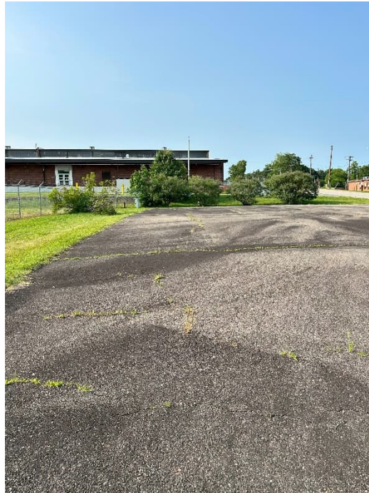
Photograph 5. OU 12 cap looking north from south end.
