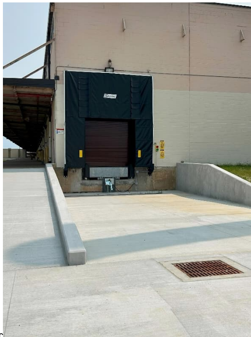
Photograph 28. Closeup view of new loading dock at northeast corner Bldg. 65.
