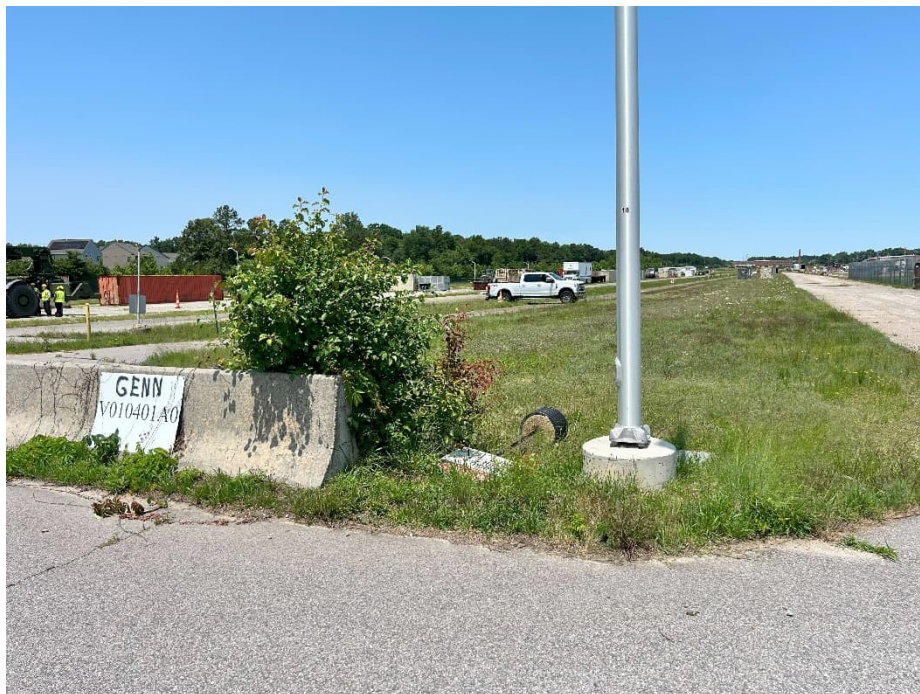
Photograph 15. Underground cable repair work in southern area of OU 1.
