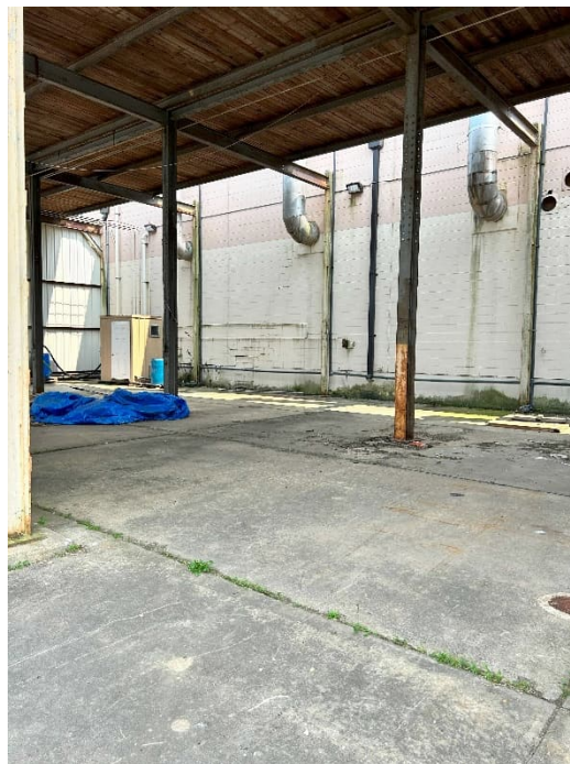
Photograph 122. Interior view of covered storage area attached to Bldg. 65, looking towards the SSDS shed.
