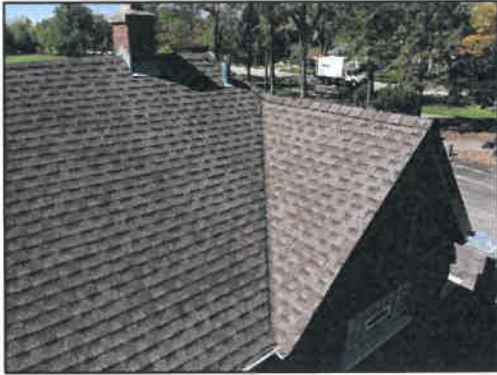
Gilbert Park Roof
