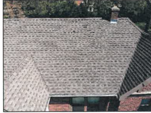
Gilbert Park Roof
