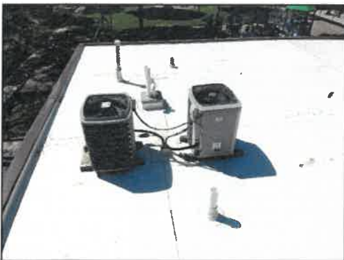
Community Center Roof
