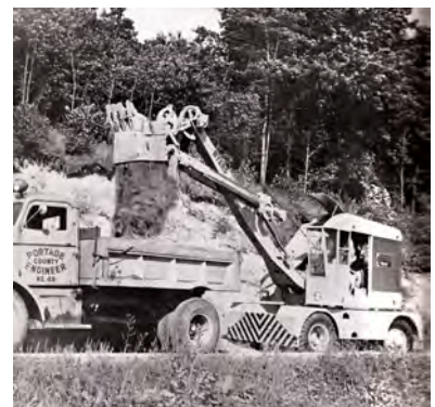
The John F. Byers Machine Company Traveler was an example of self-propelled shovels built in the 1940s. Self-propelled and truck-mounted excavators were popular for highway and road departments because of their mobility. (Byers brochure 1248, 1948)
