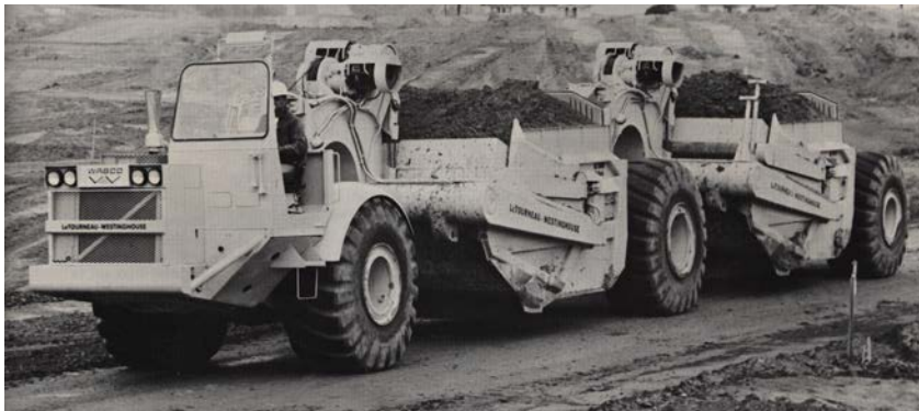
A LeTourneau-Westinghouse C-500 prime mover with two unpowered scrapers.
