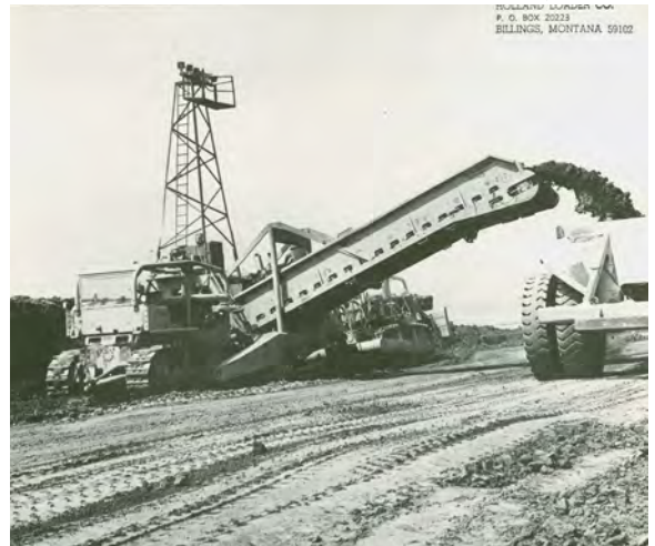
One of the four Holland loaders at Perris Dam makes quick work of loading a 110-ton capacity Euclid bottom dump. It's equipped with a vertical cutting edge.
