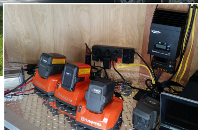
A look at the battery charging station inside a model solar-equipped trailer (with solar panels on top of trailer).
