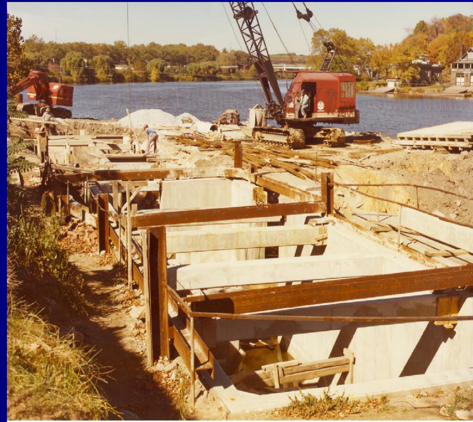
Construction Of Fairmount Fish Ladder, 1978
