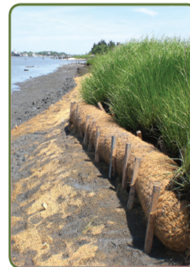
A coconut fiber log is deployed along the edge of a tidal marsh in Bivalve, New Jersey, in an effort to establish a "living-shoreline" reef that may soon protect against erosion.
