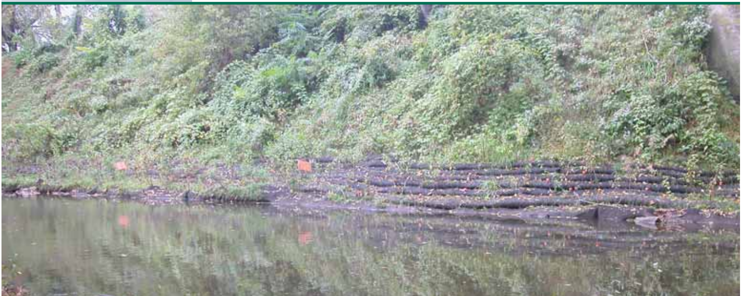
Vegetated erosion control tubes protect Stony Creek from bank erosion
