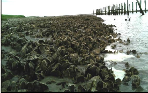
Oyster/Rock Breakwaters
