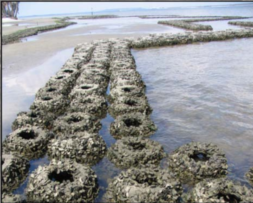
Oyster dome breakwater
