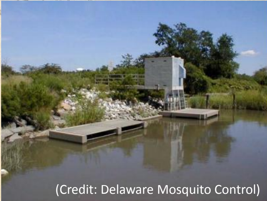
Broad Dyke Marsh water control structure
