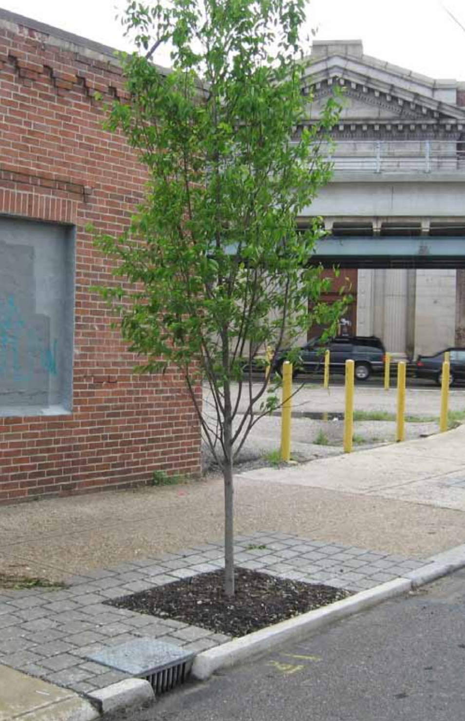
Norris Street Stormwater Tree Trenches, Philadelphia
