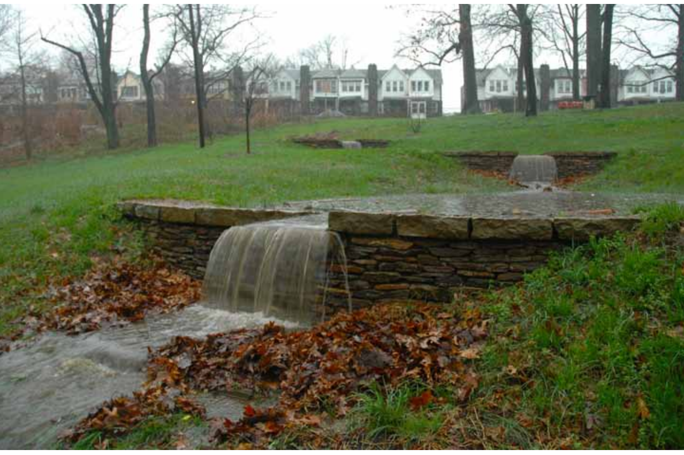
Cliveden Park step pools during a rain storm
