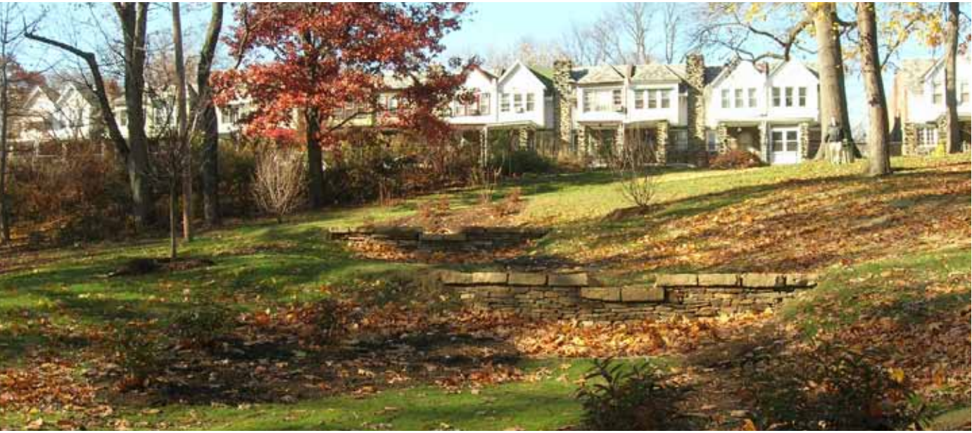
Cliveden Park step pools during dry conditions
