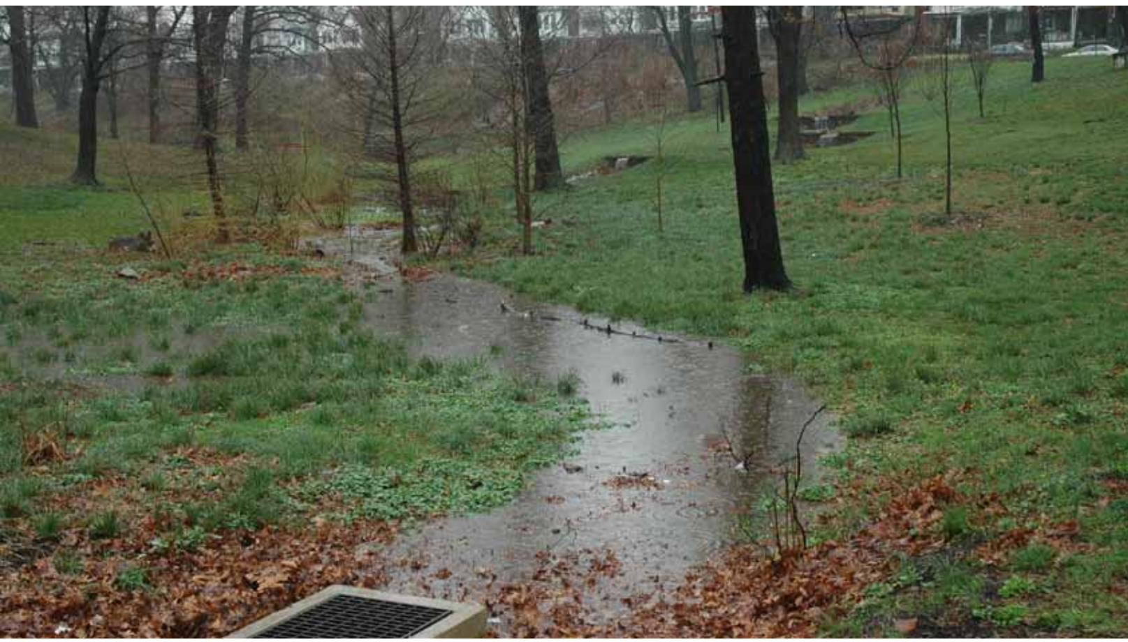
Cliveden Park swale during a rain storm
