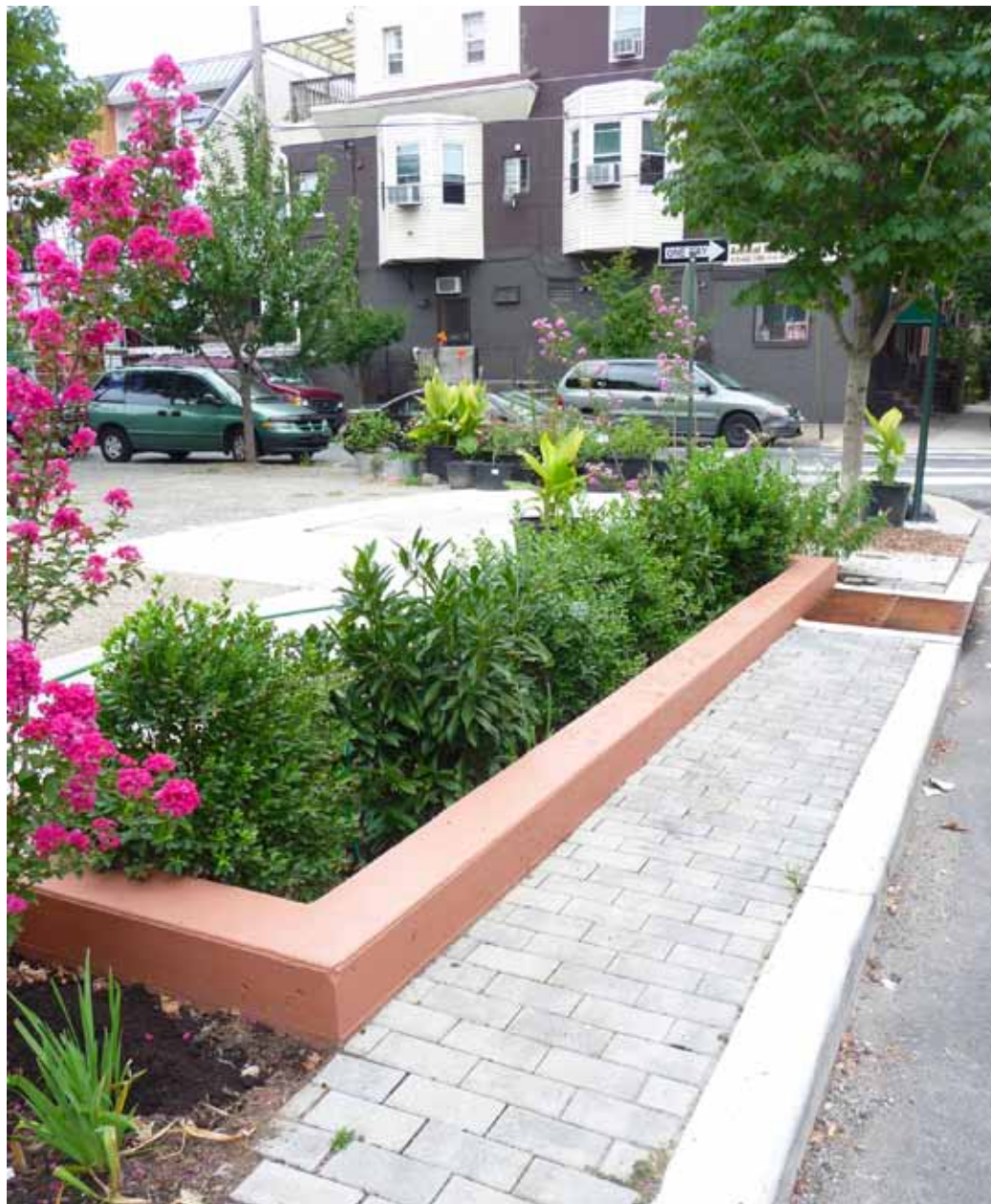
Columbus Square stormwater planters, Philadelphia
