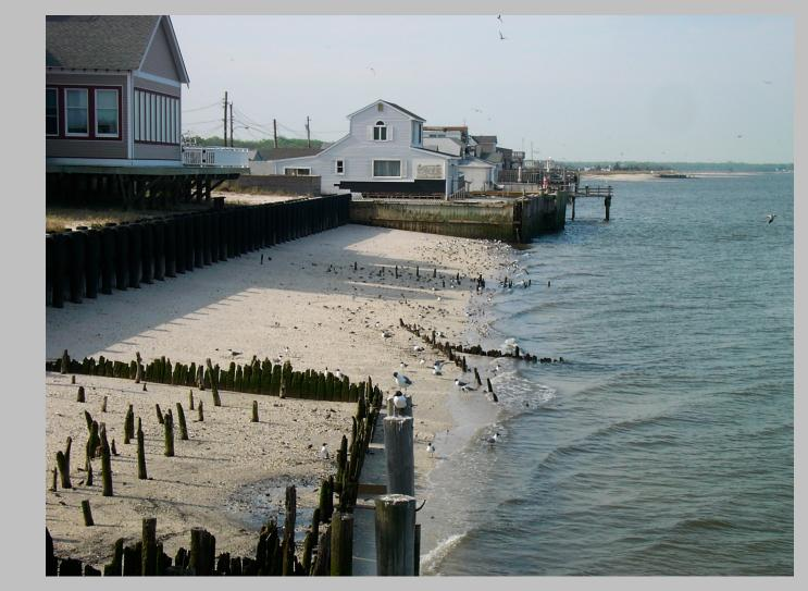
Many bulkheads are built incrementally over time and intersect the shoreline at different elevations.
