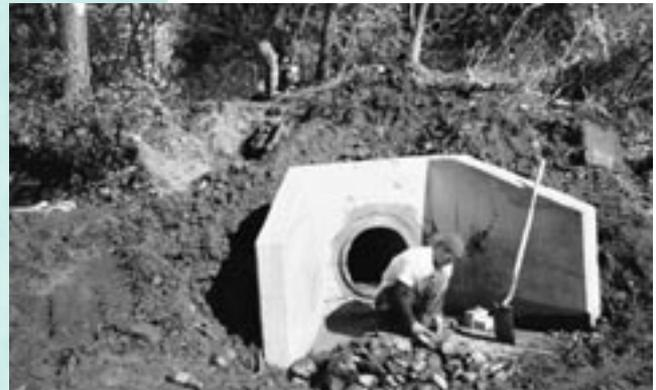
*"Working on Headwall" -- A worker has placed special cement that hardens even in wet environments and is placing rocks around the back of the headwall. A wall of dirt on the inland side of the pipe has not yet been removed to allow water to flow through the pipe.*
