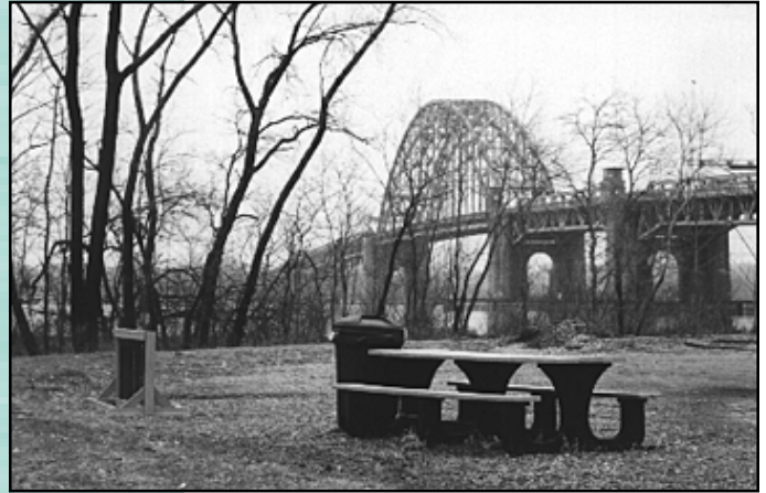
View of the Tacony-Palmyra Bridge from the Palmyra Cove Nature Park in Burlington County, New Jersey
