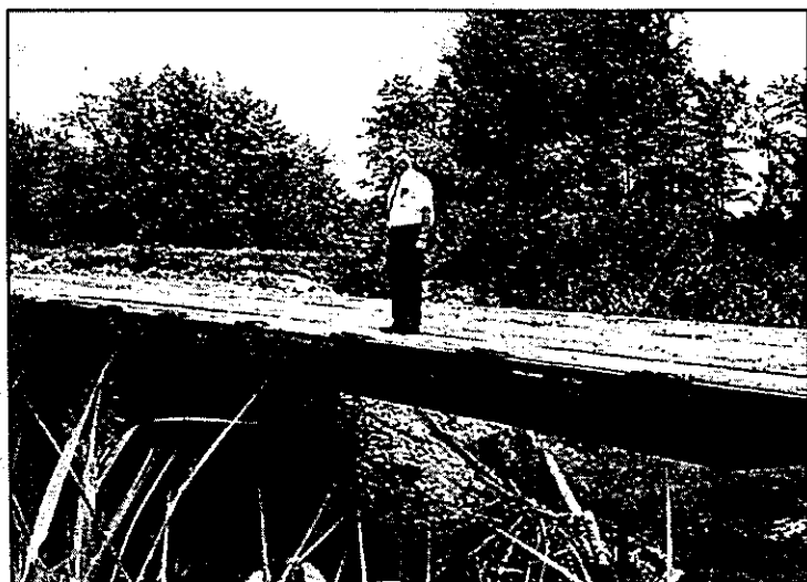
RECYCLED FLATBEDS — Ballard County Judge-Executive Bill Graves stands on the new railroad flatbed bridge on Goose Haven Road in Oscar, Ky., Tuesday. Two flatbed cars destined for the scrap yard were converted into the bridge, to save taxpayers thousands of dollars.
