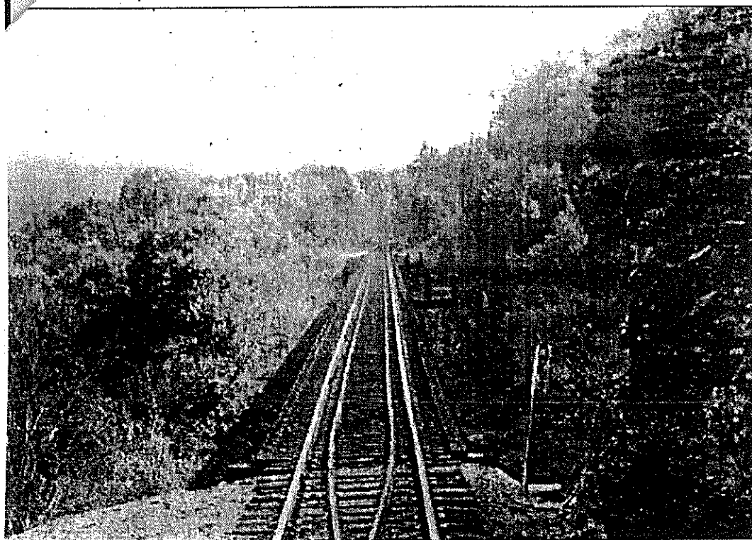
Trestle #3 along the way to Van Buren.
