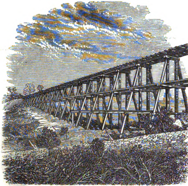
No. 1. Trestle opposite Auburn.
