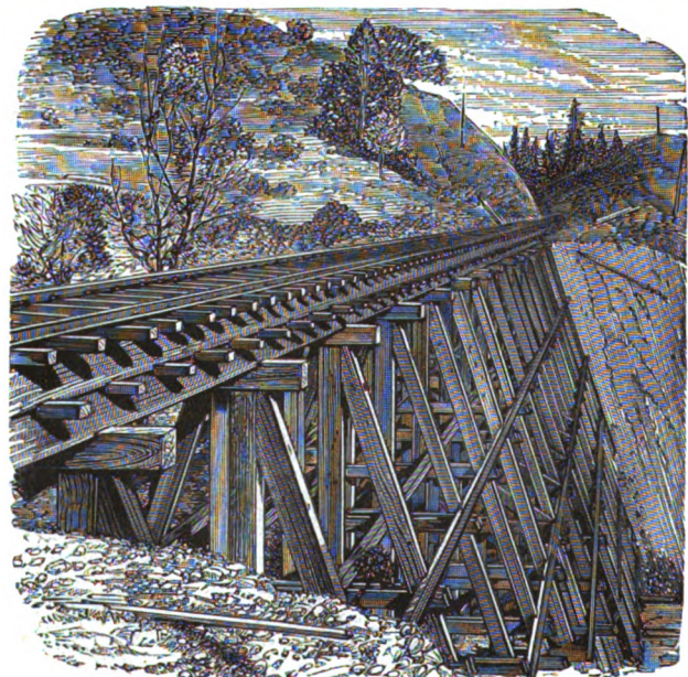
No. 6. First Trestle in Clipper Ravine.
