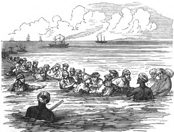
Landing the Indo-European Telegraph Cable in the mud at Fao, Persian Gulf.
