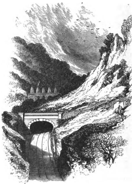
LAND-SLIP ON NORTH MIDLAND LINE. NEAR AMBERGATE.
