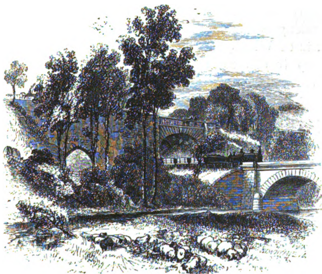
BULL-BRIDGE, NEAR AMBERGATE.
