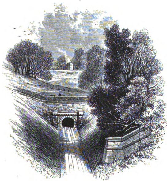
KILSBY TUNNEL. [North End]
