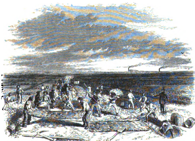
CHAT MOSE—WORKS IN PROGRESS
