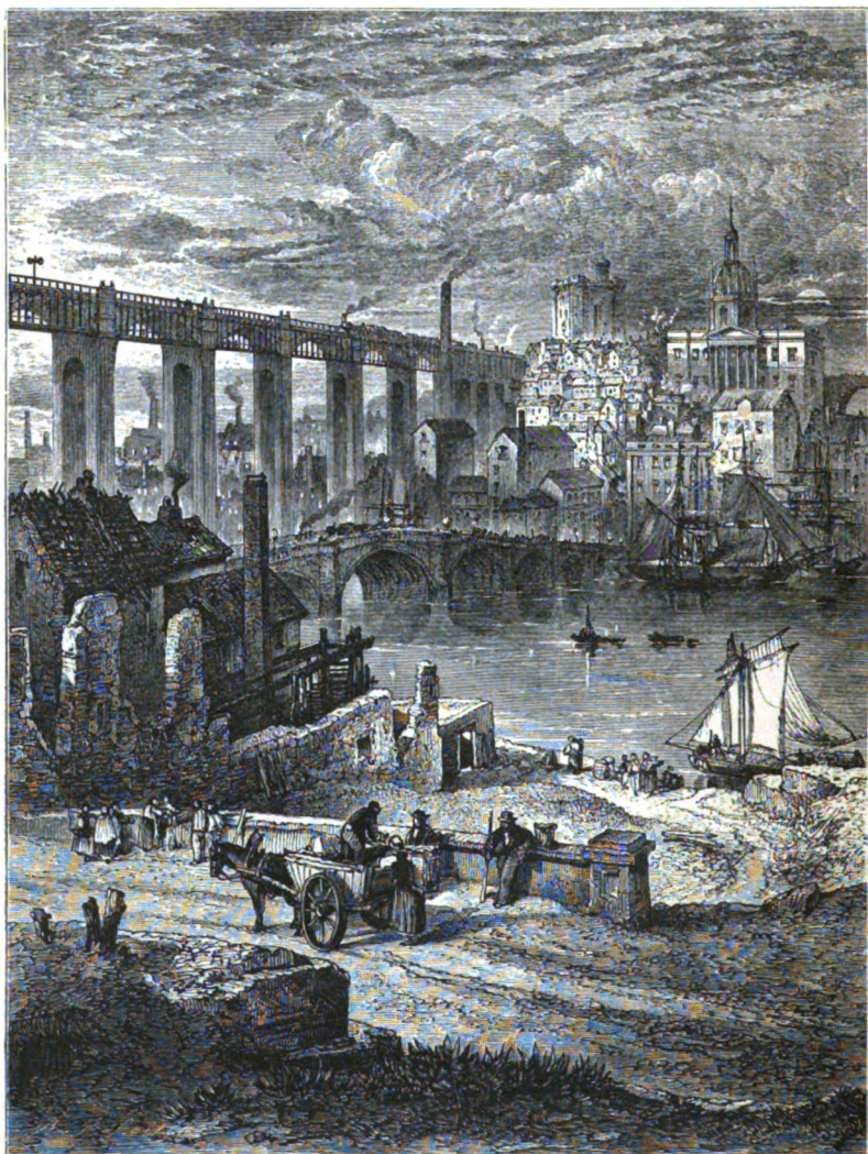
NEWCASTLE-UPON-TYNE AND THE HIGH-LEVEL BRIDGE.
