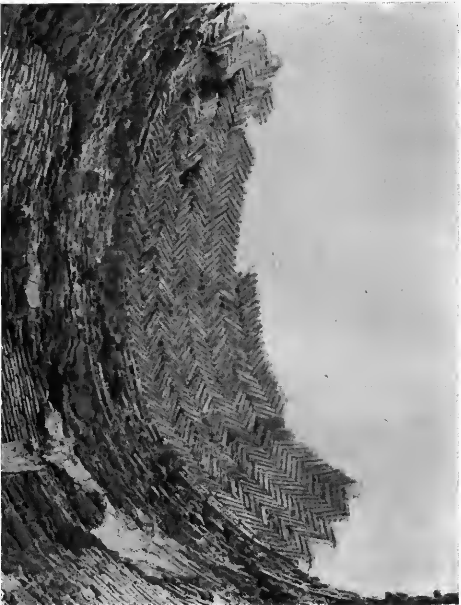
109. Tomb of king Faceh Khan's sister. Interior view of gulf collapsed dome showing bricks used in zigzag pattern for strength as well as to construct curved surface.
