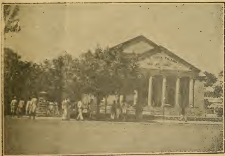
View from the North-West.
