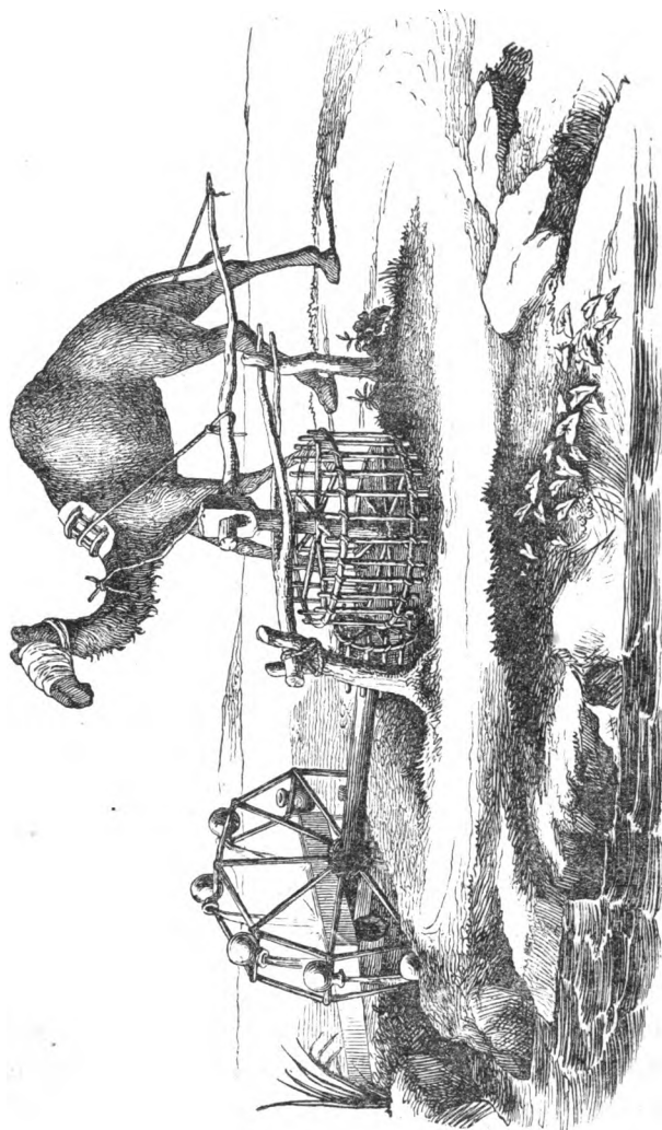
PERSIAN WATER-WHEEL WORKED BY A CAMEL.
