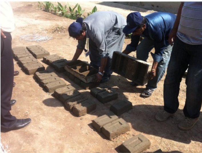
Ar. Phulpoto and Ar. Domki making mud/adobe bricks.
