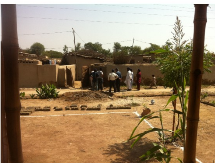
Demonstration of application of mud-lime plaster.
