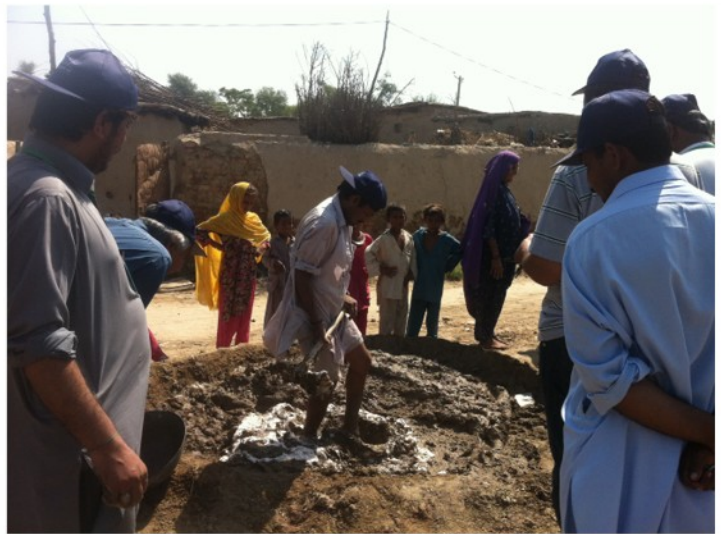
Mud-lime mix for plaster being prepared.
