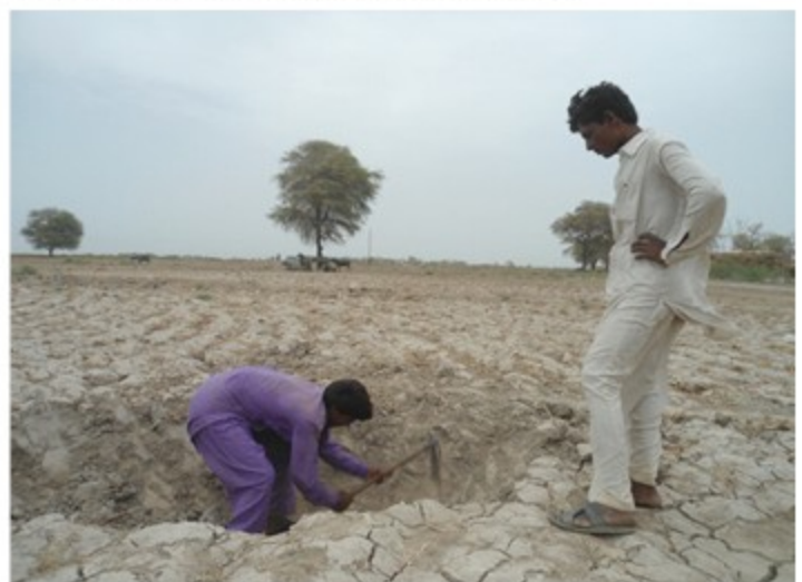
Digging for foundation at Ghuram Bhatti village, Mirpur Khas
