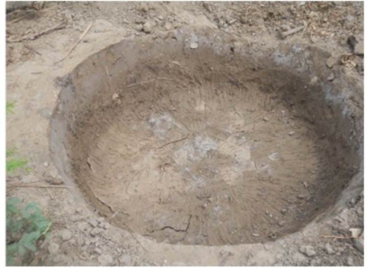
Lime pit preparation at Qazi Noor Ahmed Village, Mirpur Khas
