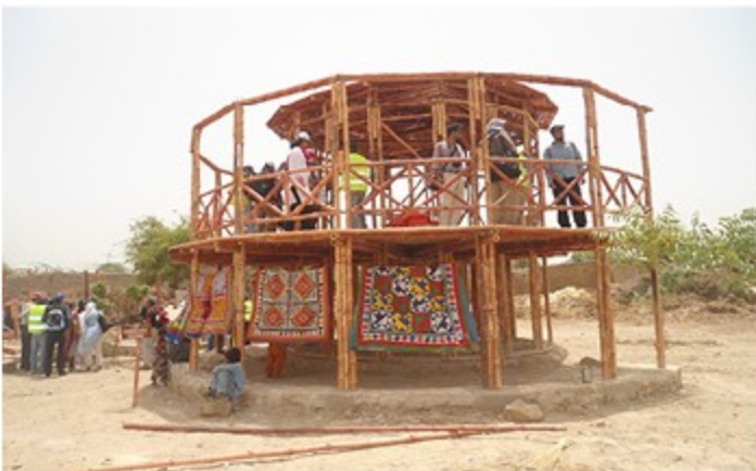
Community Centre construction in bamboos
