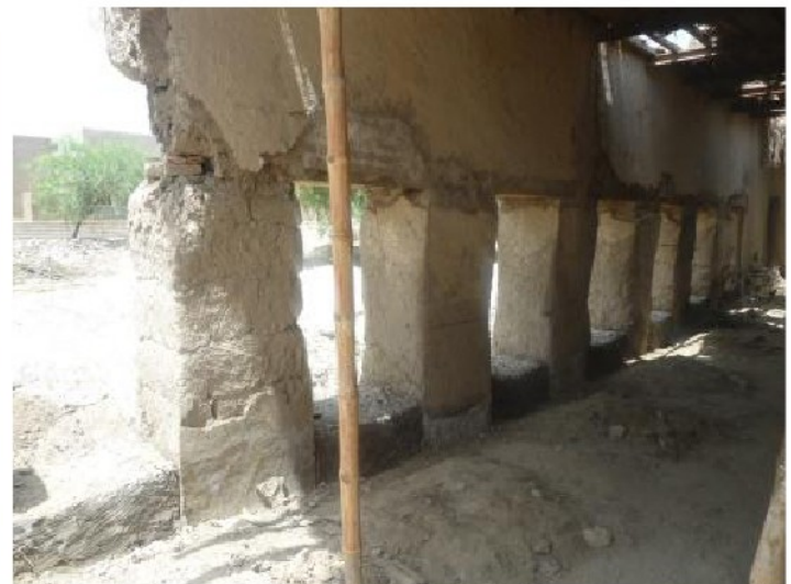
Ongoing stabilization of the veranda columns
