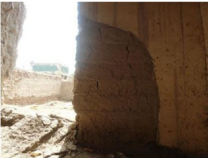
Stabilization of an exterior wall, using Mud bricks
