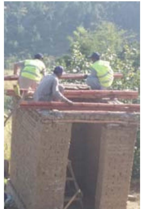
Learning about bamboo jointing and placing bamboo joists on roof.
