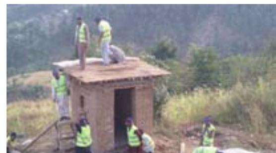
Completing the roof for receiving water proof layer of lime pozzolana.
