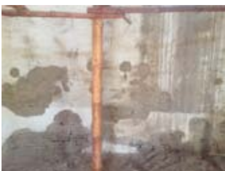
Filling open mortar joints at the base of walls
