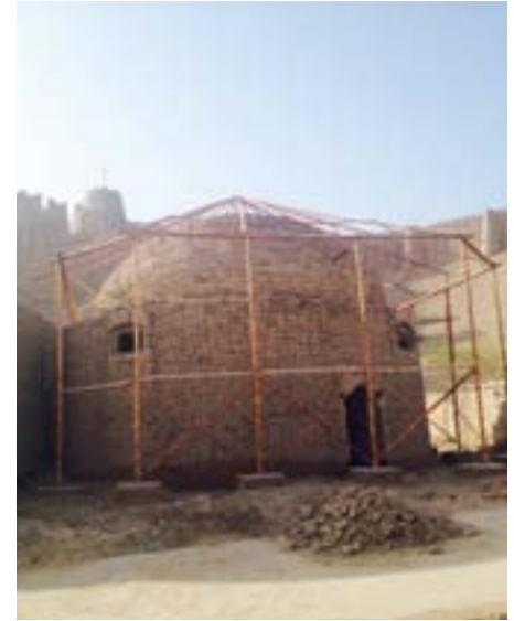
Erection of scaffolding
