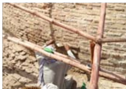
Pointing of mortar joints.
