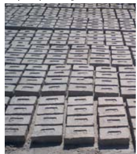
Fabrication of bricks for retaining wall
