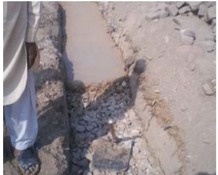
Construction of Retaining wall
