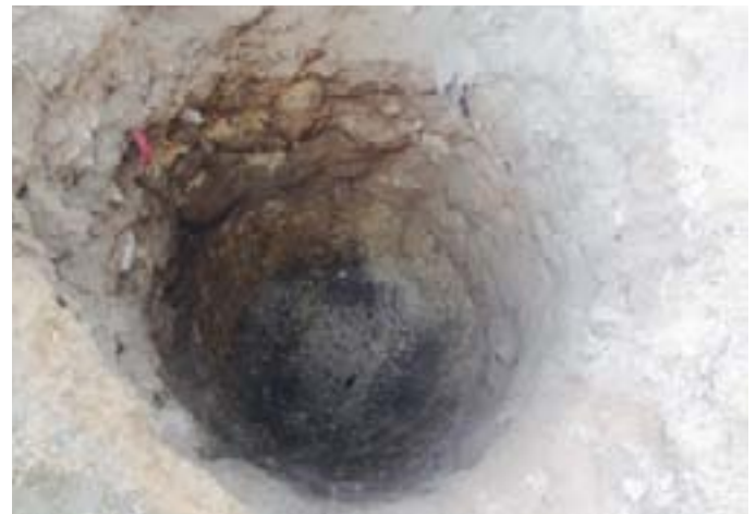
Excavation of pit to investigate depth of water table
