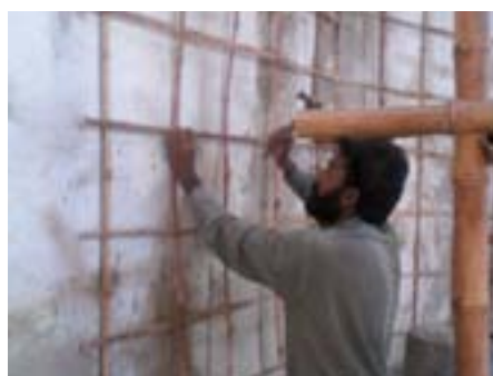
Fixing bamboo lattice to internal walls
