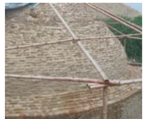
The structure remains unharmed.
