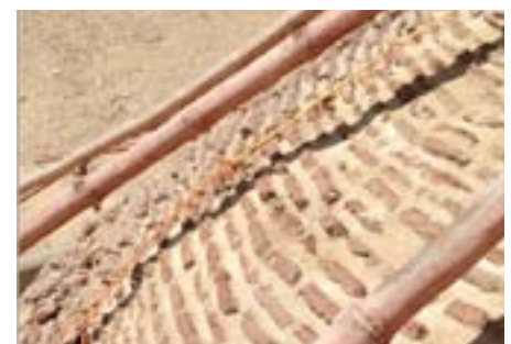
Completed filling of mortar joints on the dome.
