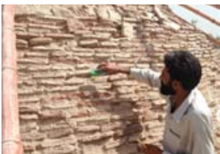
Dry cleaning before the pointing of mortar.
