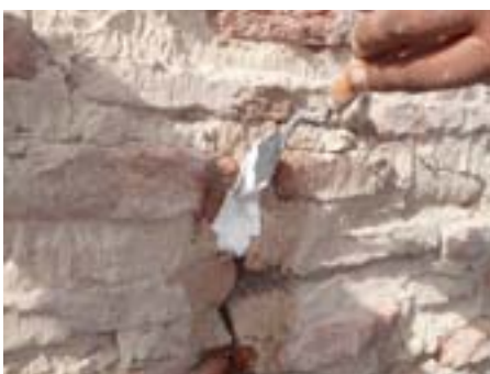
Filling cracks with lime, gypsum and brick dust
