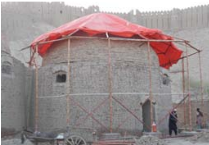
Installation of tarpaulin for temporary protection from rainwater
