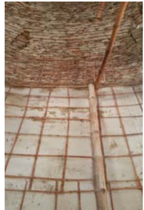
Bamboo lattice on internal masonry on 5.3
