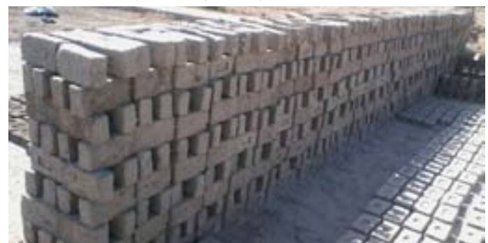
Fabrication of bricks for retaining wall
