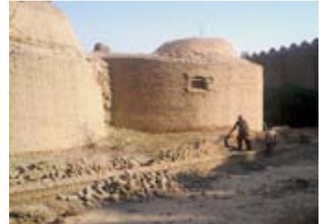
Construction of Retaining wall
