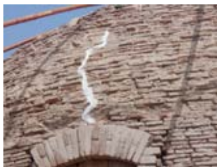
Filled cracks in dome
