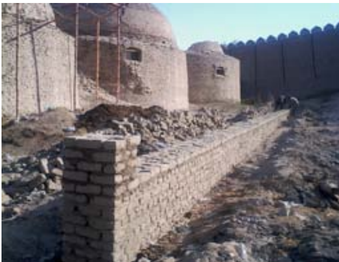
Construction of retaining wall
