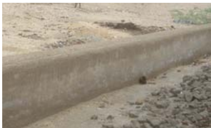
The wall around the granary to provide protection against gushing rain-
