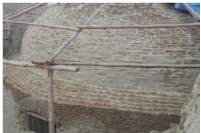
All the voids were filled and further covering of the tarpaulin.
