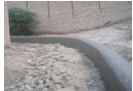
Construction of Retaining wall completed
