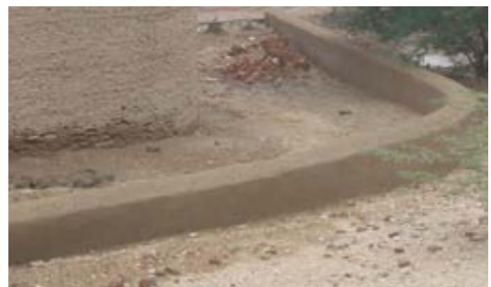
Rain water prevented from collecting by the wall around the granary.
