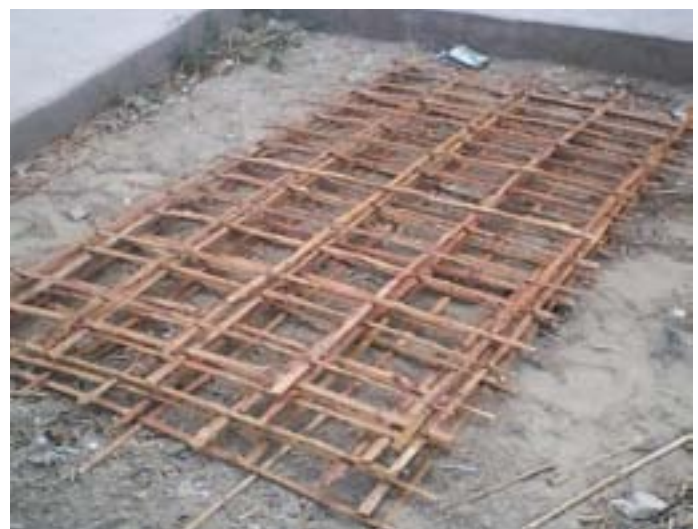
Bamboo lattice prefabricated for installation inside granaries
