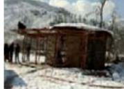
Based on the bamboo cross bracing developed for the Zero Carbon Footprint house in Swat, a Green Women's Centre was built in village Beha in Matta in an area that had been wrecked by militants. This was the first bamboo roof with a span of 16' and it was tested the same year when the snow piled up 3' to 4'. This was also the first centre that was built for women. Later a few more centres were built by the Foundation in order to provide socializing and working space for women in Swat.
