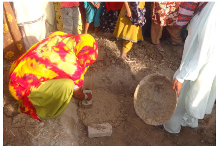
Demonstrating laying of PLC layer during Practical Field work session
