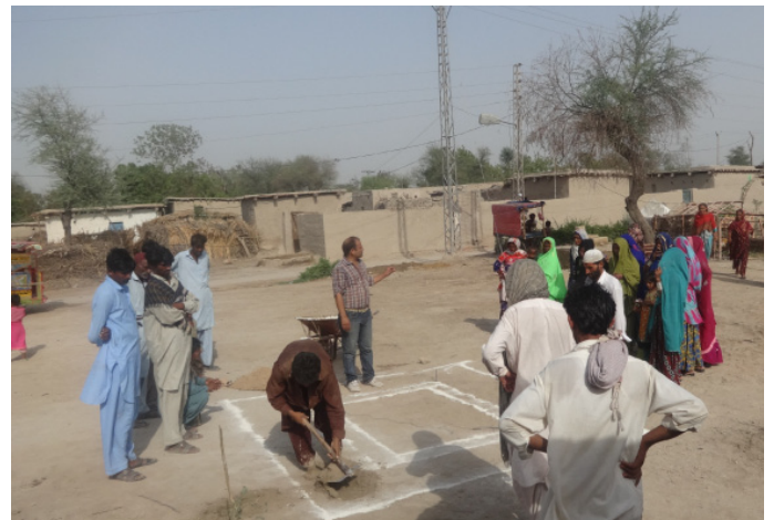
Layout and excavation demonstration of the Latrine
