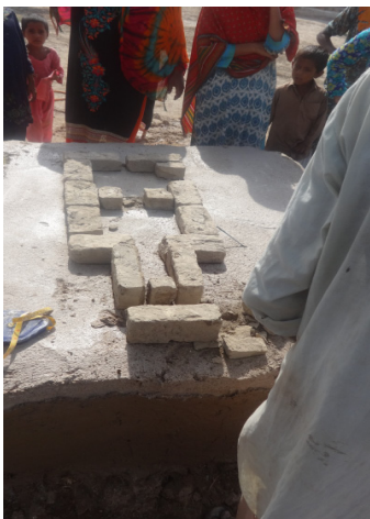
Constructing the Chulah
