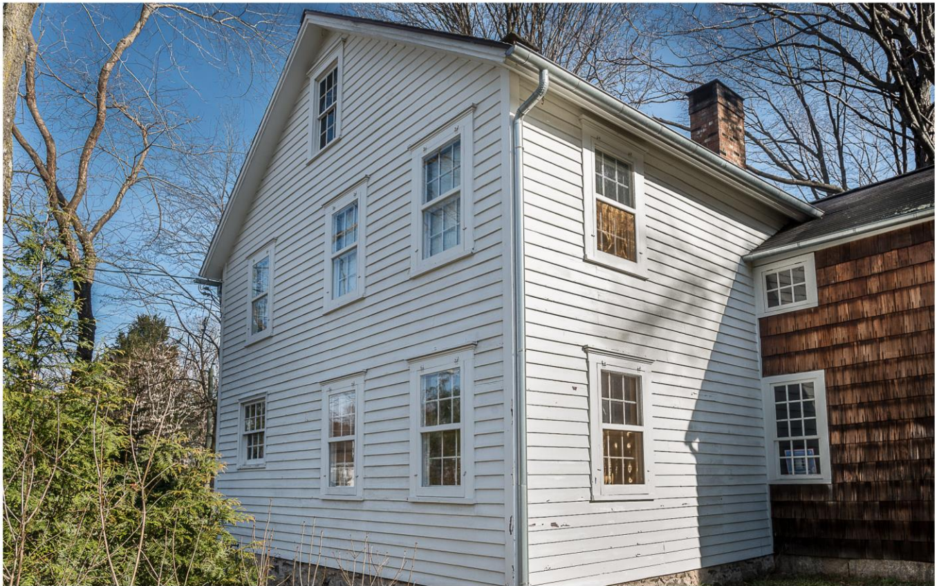
Photo 3. View northeast showing west and south elevations of nineteenth century addition.
