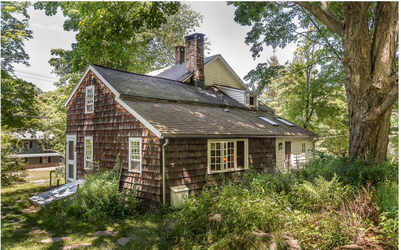
Photo 6. View northwest showing facade of original block and east elevation with leanto.
