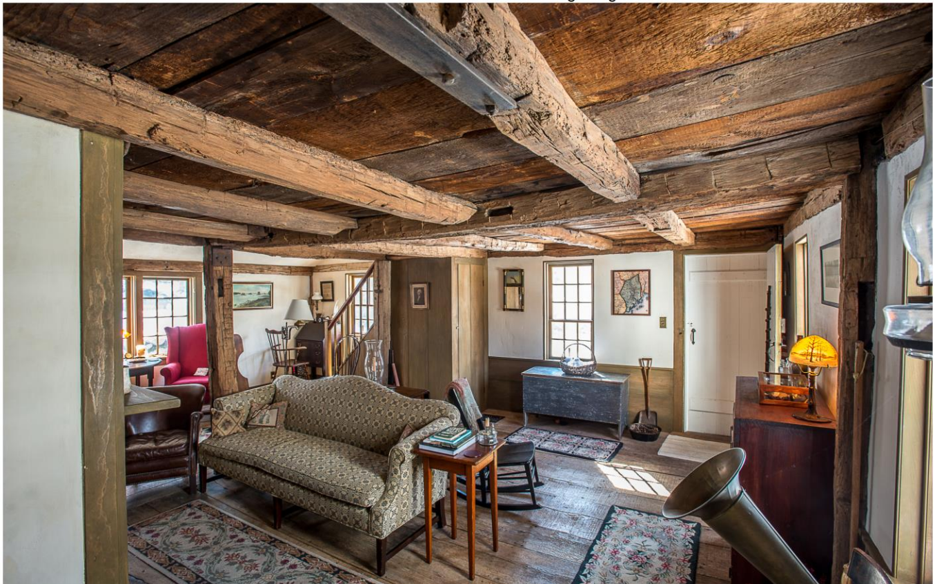
Photo 16. Interior view southeast showing living room.
