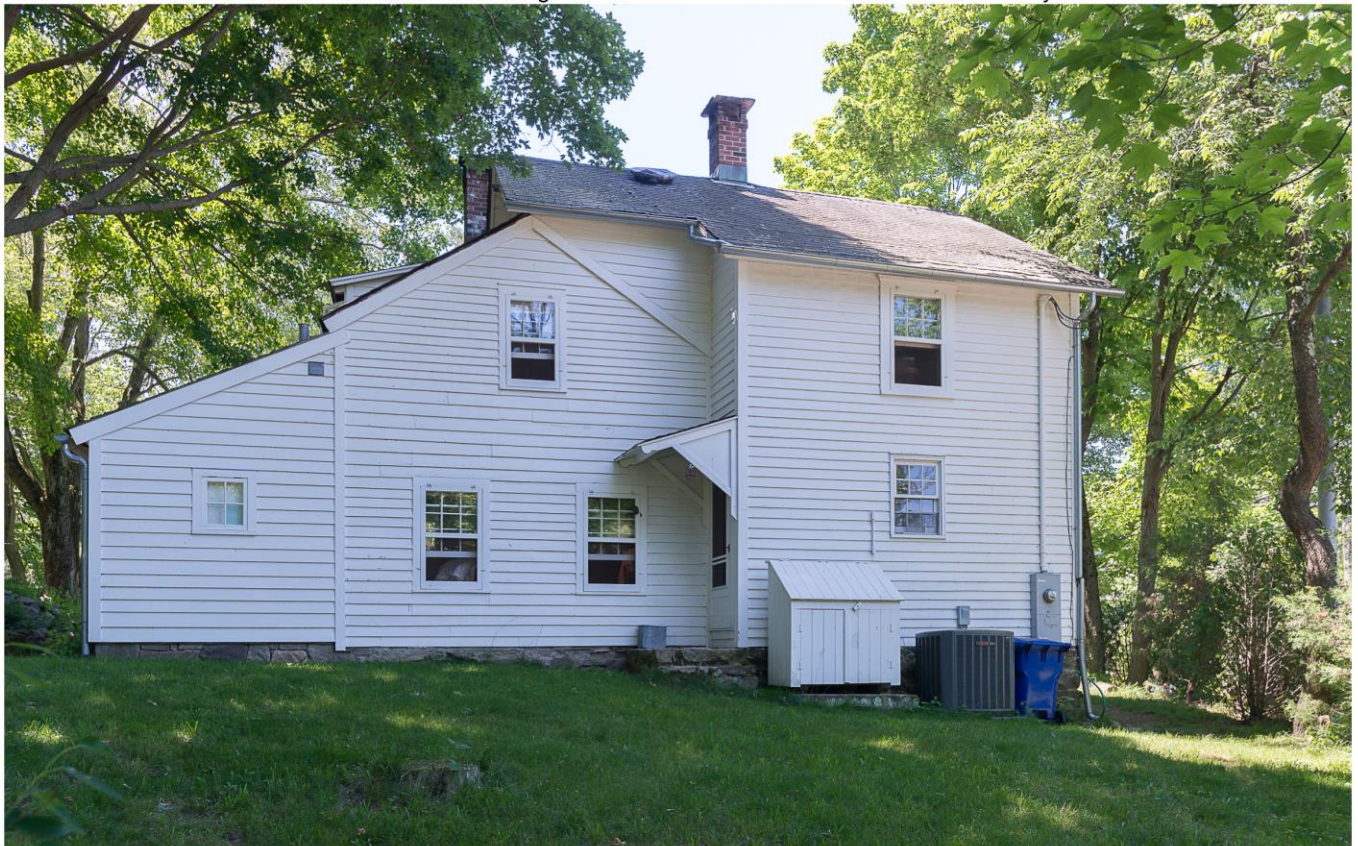
Photo 4. View south showing north elevation.
