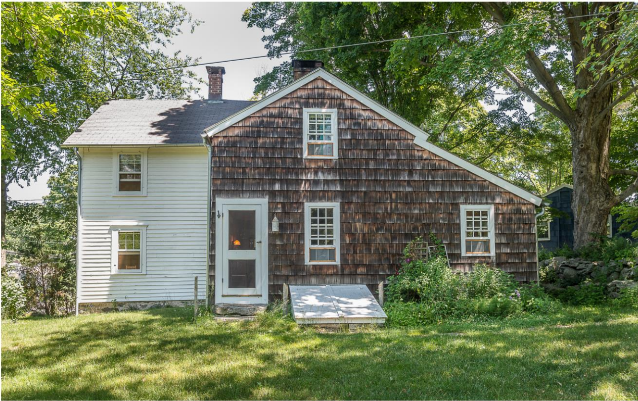
Photo 1. View north showing facade of original house and south elevation of nineteenth century addition.
