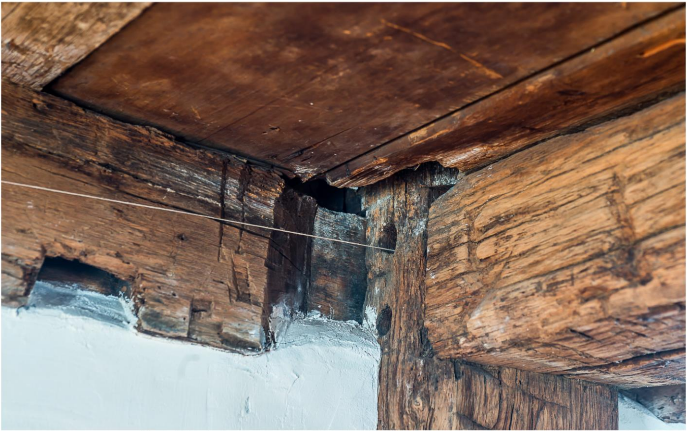
Photo 27. Interior view northwest showing joints in timber frame on first floor.
