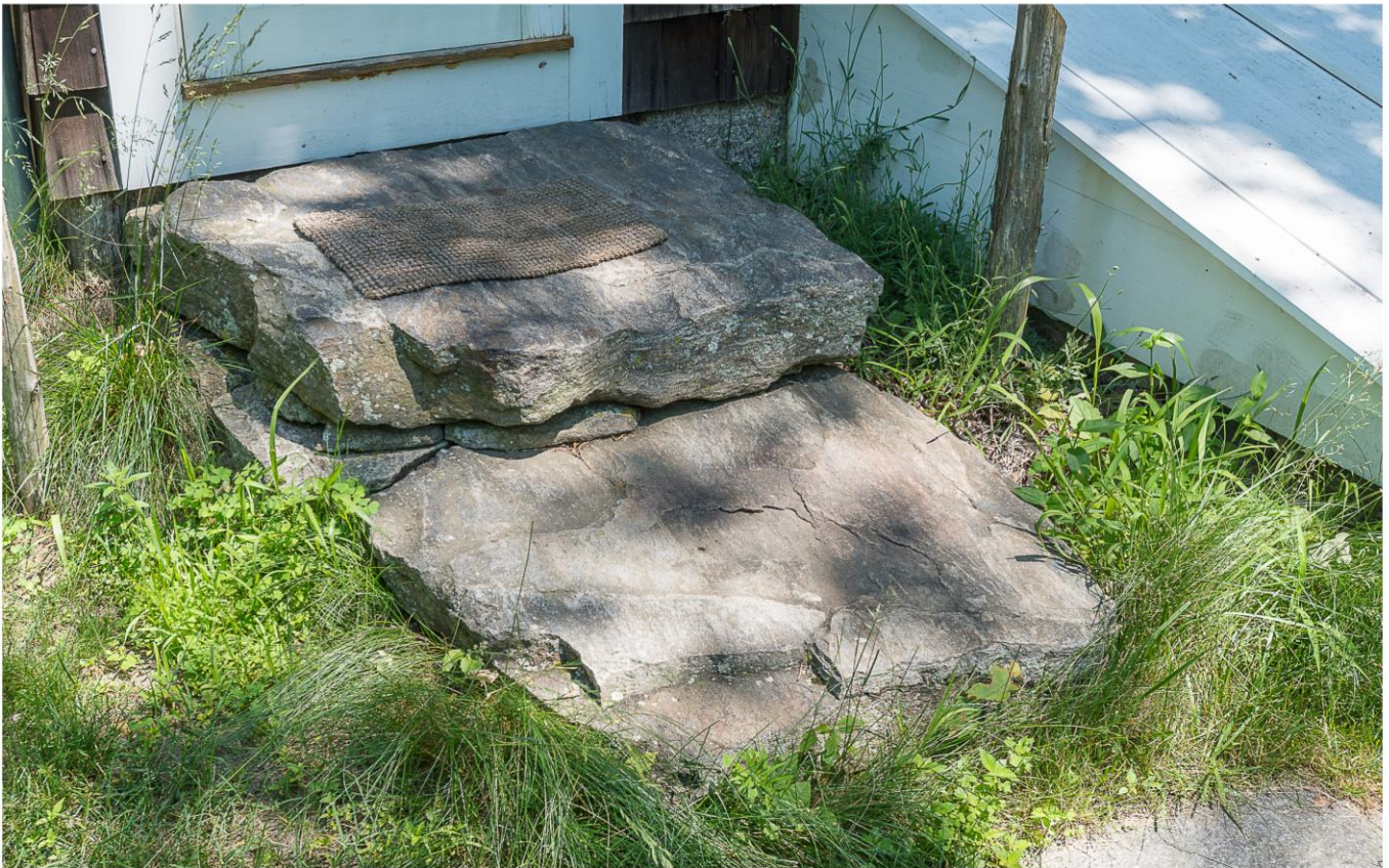
Photo 7. view northeast of stepping stones leading to main entrance.
