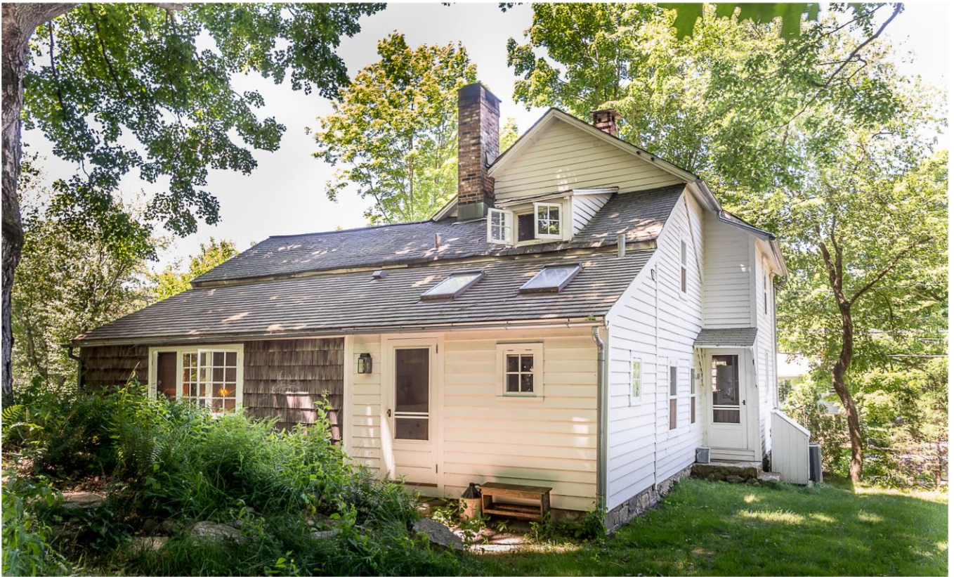
Photo 5. View southwest showing east elevation and part of north elevation. Eighteenth century section is covered in unpainted shingles and nineteenth century section is covered in painted clapboard.
