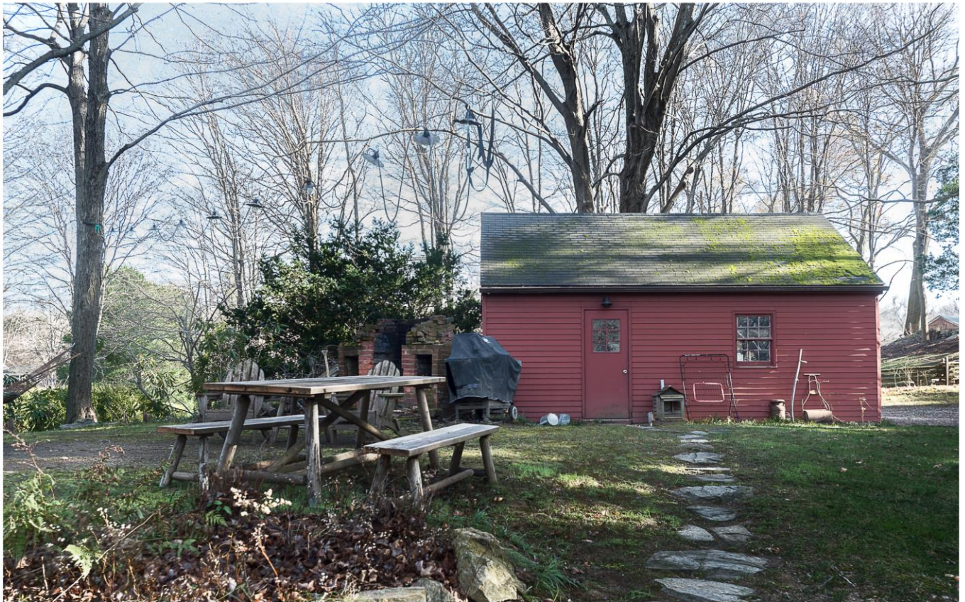
Photo 11. View east showing west elevation of garage.
