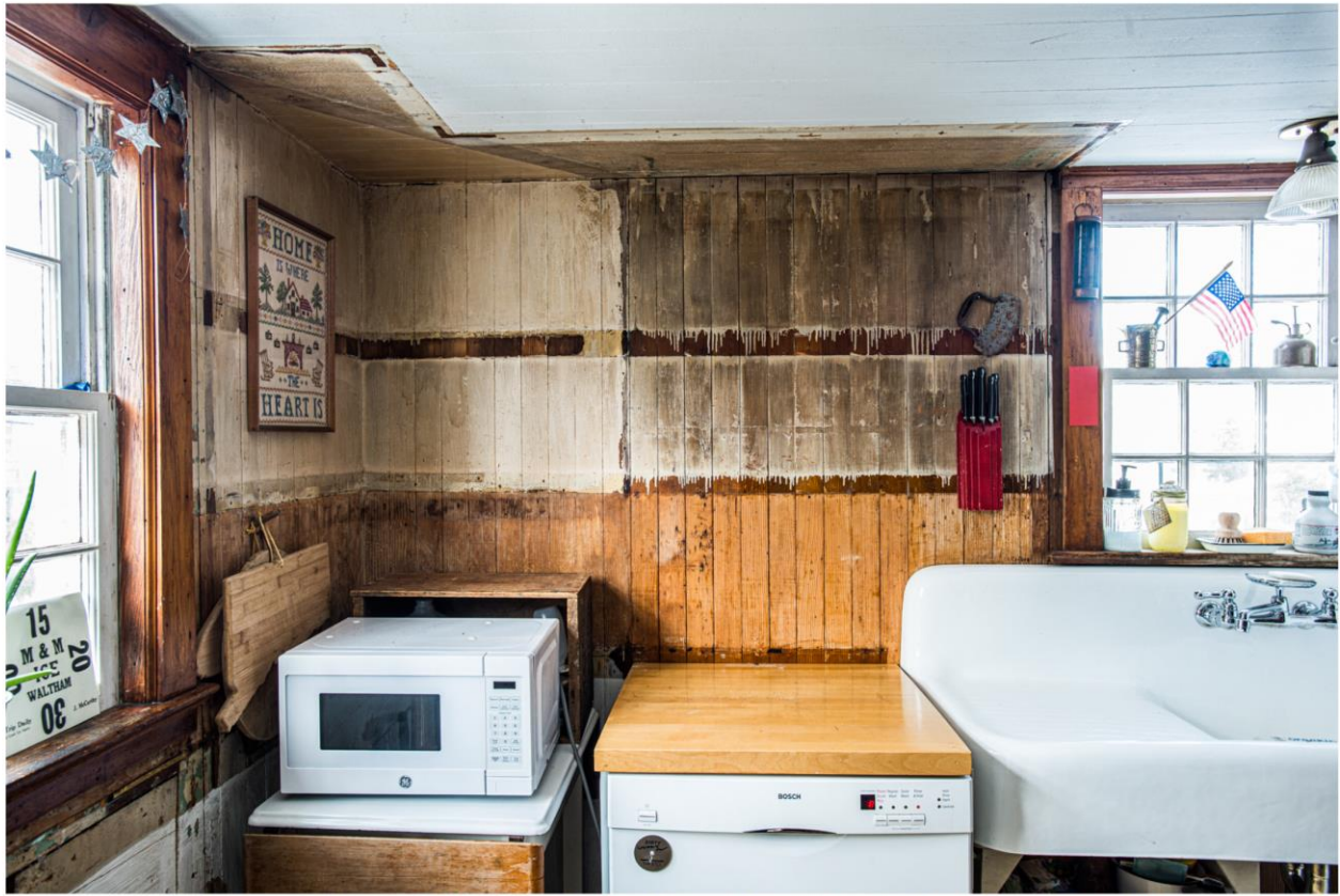
Photo 19. Interior view north of kitchen showing vertical strip ash walls and section of ceiling.
