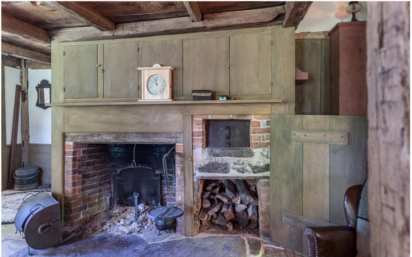
Photo 13. Interior view northwest showing main fireplace.
