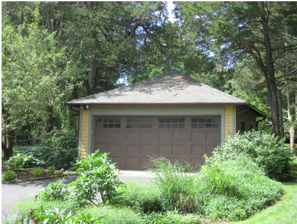
8. East view of the garage. Camera facing west.
