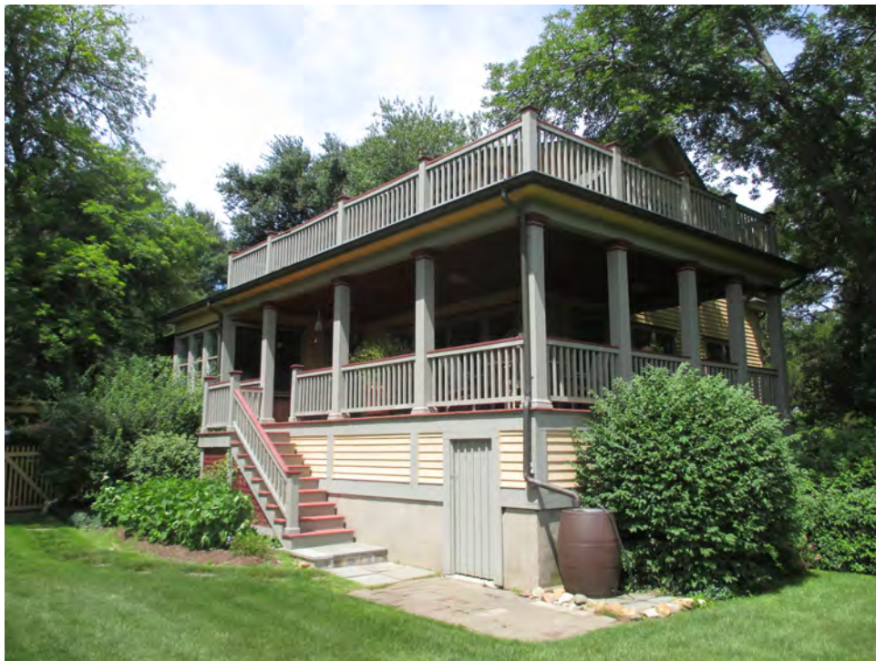
12. South elevation and east elevation of the house. Camera facing northwest.
