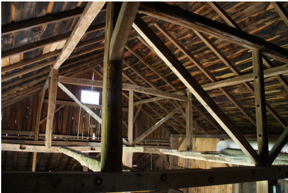
12. Interior view of English barn, camera facing west. Note the hand hewn timber frame with dropped tie-girts, queen post trusses, and purlin plates.
