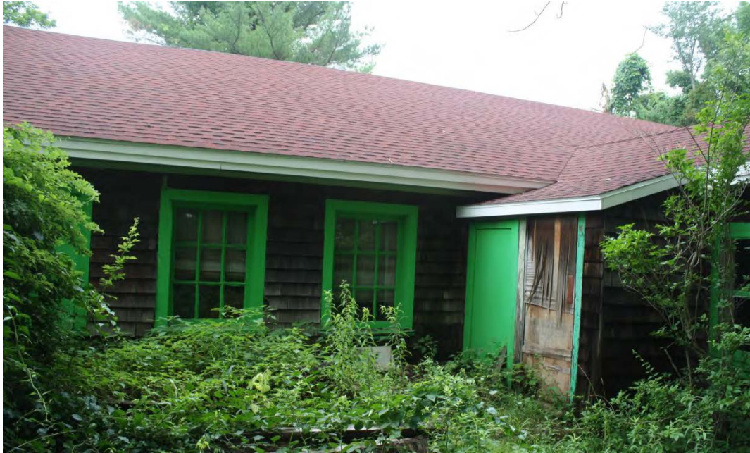
10. East detail view of Barn/studio, camera facing west. Note nine=pane dairy barn windows and attached shed.
