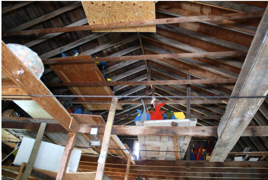
19. Interior view of Barn II; camera facing north, showing balloon frame construction.
