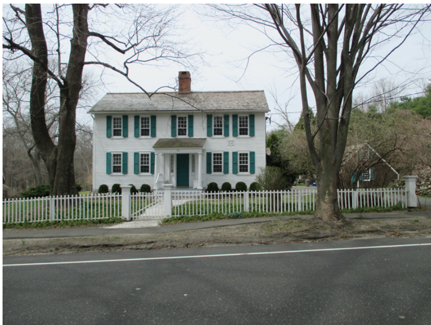
Southeast facade of the house. Camera facing northwest.
