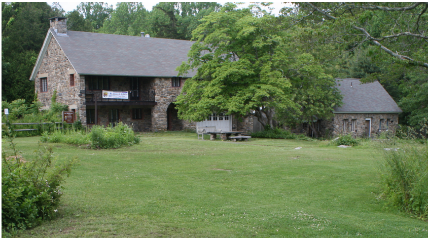
Lape-Reed and Murdock Houses, south view
