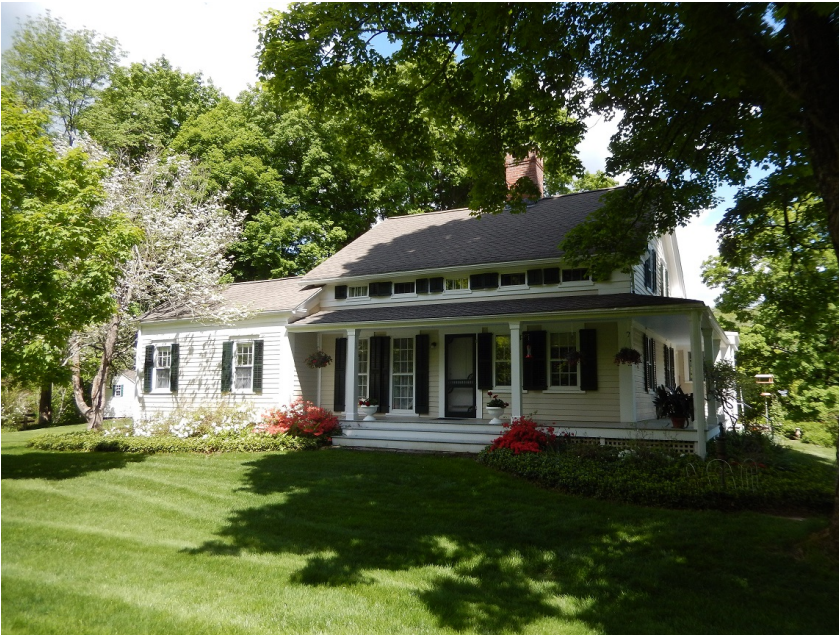
Southwest view of the house, camera facing northeast.
