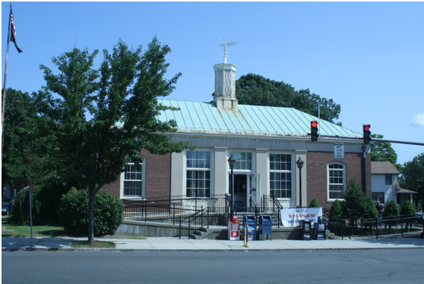
South view (facade) of the Post Office, camera facing north
