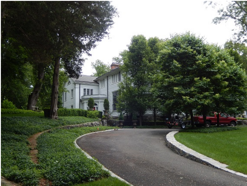
Northwest view of the house. Camera facing southeast.
